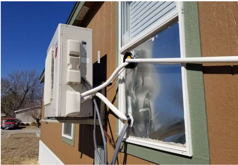
Steel window panels replaced some windows to increase load
