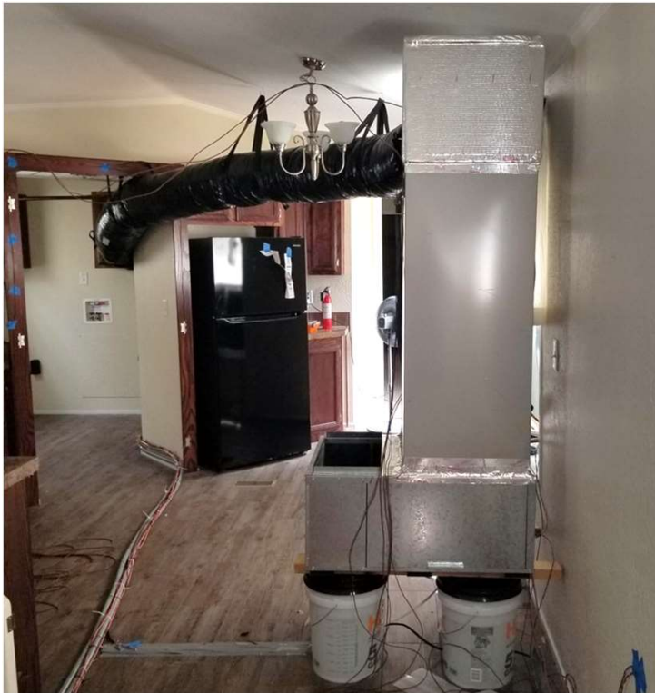
Ducted (L) and ductless (R) units installed
