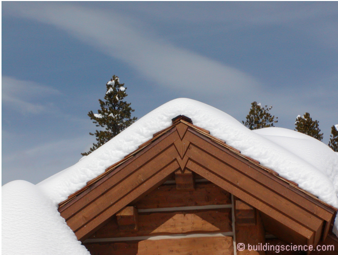
Photograph 3: Note the air inlet at the fascia. Yes, the ridge vent is covered with snow, but snow is not an air barrier. Having said that...add a “cupola” or two along the ridge to connect the “vented over roof” through the snow layer to the outside air.
