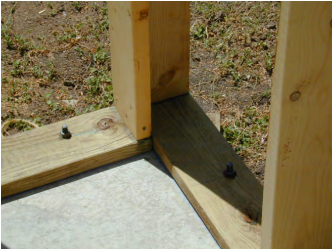
Figure 3 - Exterior Walls 2-Stud Corners
