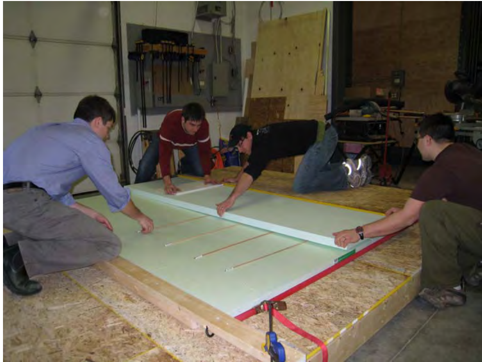
Figure 32 - Fabrication of an HDEPS Calibration Panel
