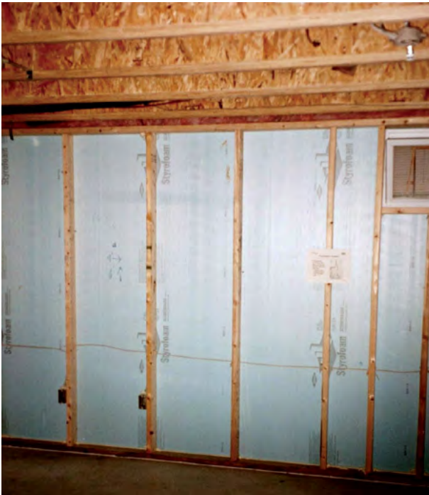
Figure: Exterior Walls 2" x 6" Studs 24" Stud Spacing
