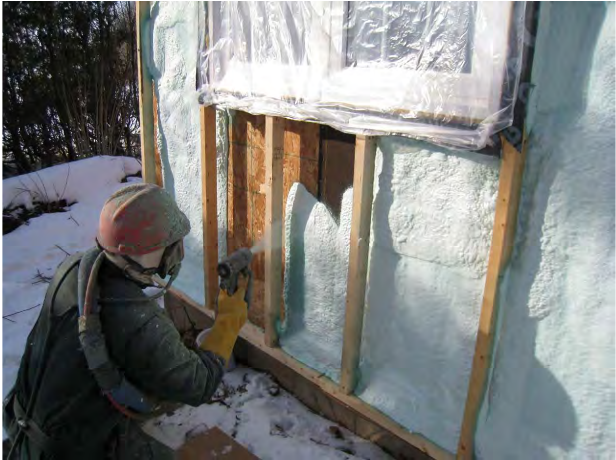
Figure 15 : Installation of high density spray foam in an Offset Framed Wall in a cold climate
