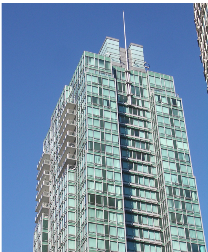
Photo 2: Almost the entire façade of this condominium tower is covered with low R-value and high solar gain curtainwall. It is almost impossible to achieve a low energy, comfortable building with this approach
