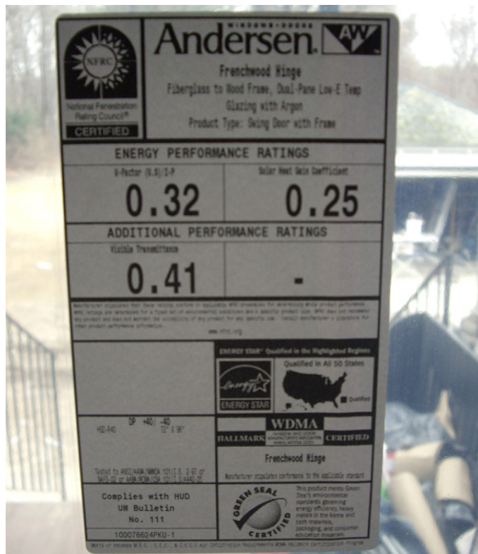
Photo 3: Residential windows usually come with an affixed sticker providing verified and useful performance values: the U-value, Solar Heat Gain Coefficient and the Visible Transmittance. Commercial window specifiers need to define these performance metrics in their construction documents
