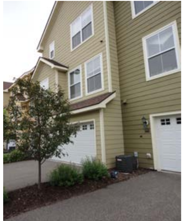
Photograph 3: Off-Set Walls - This makes the fire wall air sealing more than a little interesting.
