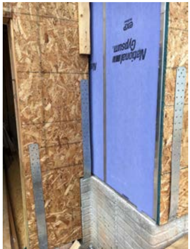
Photograph 8: More Off-Set Adjacent Units – Why do architects do this to us?
