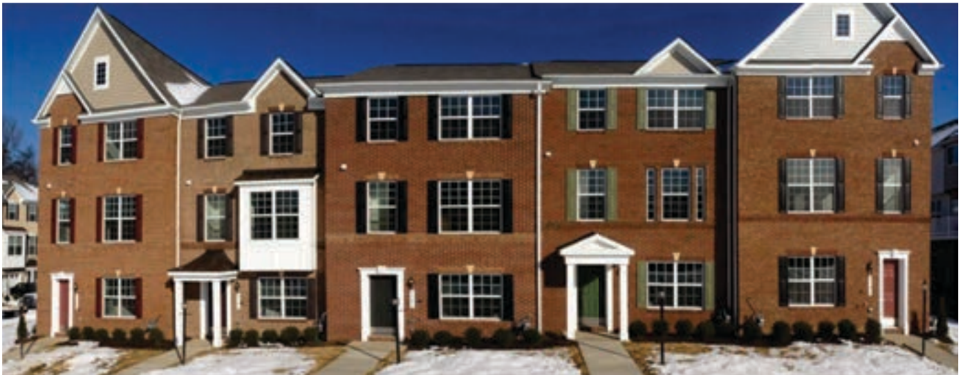
Photograph 1: Row Houses – Beautiful until you try to have them meet building code air leakage requirements.
