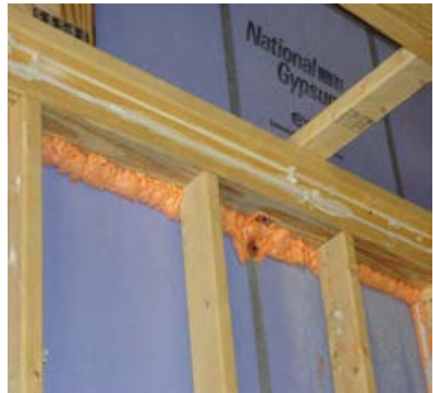
Photograph 5: Expanding Foam - Alternative way of sealing at every floor. You can use expanding spray foam. Tough to make it continuous and there is a fire load with some foams.
