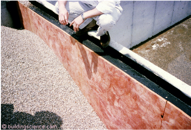
Photograph 1: Rigid Fiberglass Boards - The first real draining insulation available for use below grade was rigid fiberglass boards intended to be installed against concrete foundation walls. The oriented and layered nature of the fiberglass board made the system behave much like a thatched roof.
