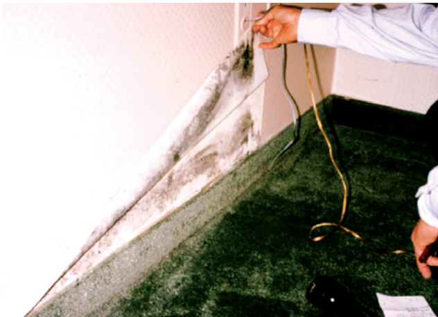
Photograph 8: Hotel Mold —Vinyl wall coverings are low perm materials that retard inward vapor movement and lead to mold growth.
