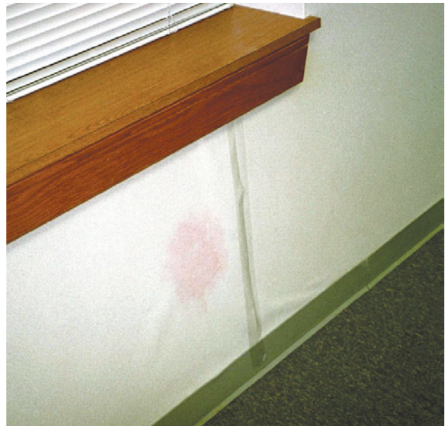
Photograph 7: Vinyl Wall Coverings and Hotels —Marriott measles, the Radisson rash, and the Hyatt hives.
