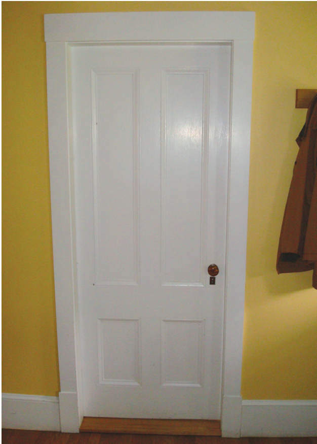
Photograph 3: Colonial Door —The most impressive “old guy” wood technology. Frames had virtually no cross-grains whereas panels which were cross-grained were allowed to slide into joints.
