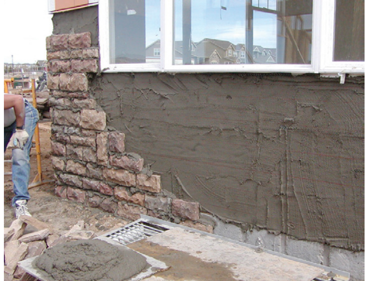
Photograph 3: Manufactured Stone Veneer —Manufactured stone veneer claddings are very similar to hardcoat stucco and perform in a similar manner. In a manufactured stone veneer the outer coat of stucco is replaced with a thin stone layer.
