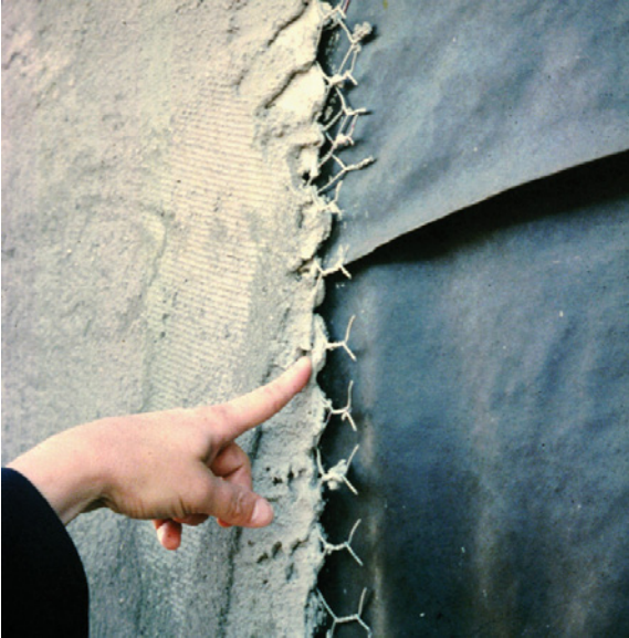
Photograph 2: Hardcoat Stucco —Three coats have been traditionally applied directly over a single layer of impregnated felt or asphalt saturated kraft paper. Today, this results in a bond between the stucco rendering and the outer layer of the felt or paper compromising drainage.
