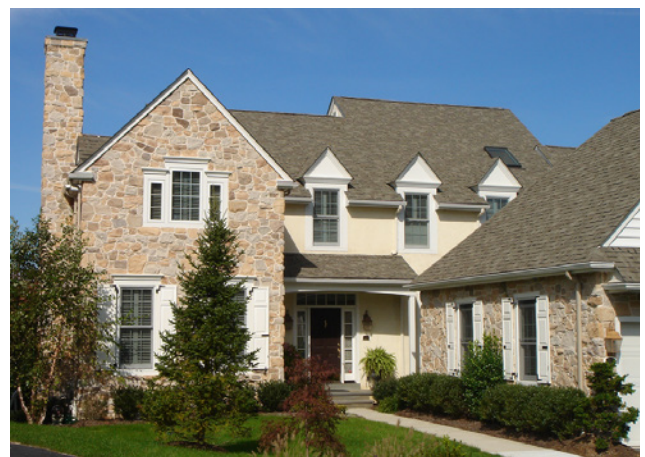
Photograph 1: Pennsylvania Stucco “Shack” —Eastern Pennsylvania is the stucco failure capital of the United States. Note the manufactured stone veneer—or “lumpy” stucco on the front façade.
