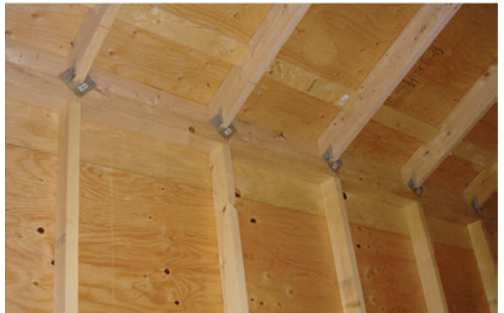
Photograph 5: Interior Structural Frame —The wood-frame wall cavities and wood rafter roof cavities remain uninsulated to control cavity condensation. The cavities provide space for services. The air barrier membrane and vapor barrier membrane are exterior to the wall and roof framing.
