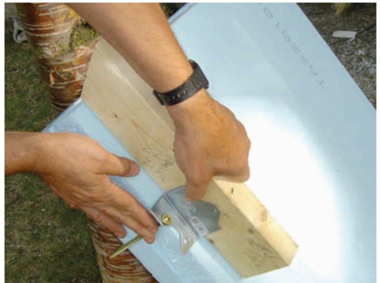
Photo 3: Ventilation Rafter —The 2x4 (standing proud) is connected through the roof rigid insulation with a metal bracket and a long roofing screw. You can purchase 14 in. (356 mm) long epoxy-coated steel screws. Stay away from stainless steel screws because the heads twist off. Stainless steel tends to be soft. Ask me how I know.
