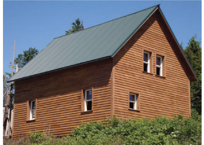
Photograph 1: Extreme Enclosure —“Superinsulated” does not do justice to this house constructed by the Hydaburg Tribe in Alaska that is ultra-airtight and ultra-vapor tight (less than 0.5 ach at 50 Pa [0.20 in. w.c.] and less than 0.5 perms).
