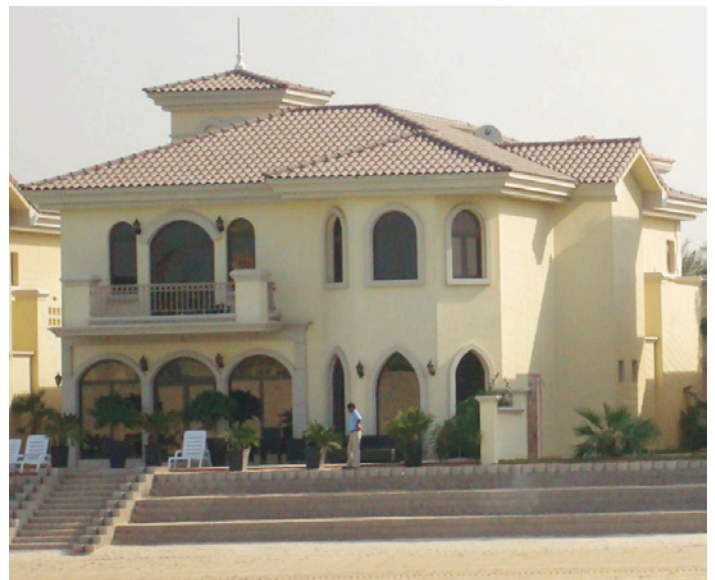
Photograph 2: Dubai Home —Stucco, tile roof, in a subdivision on a man-made sandbar in the middle of the Persian Gulf surrounded by desert.
