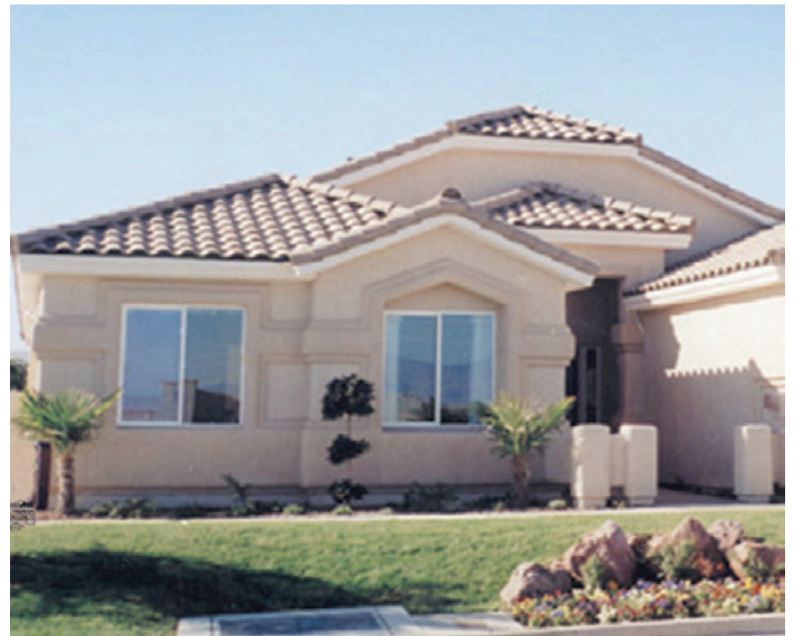
Photograph 1: Las Vegas Home —Stucco, tile roof, in a subdivision in the middle of the desert.
