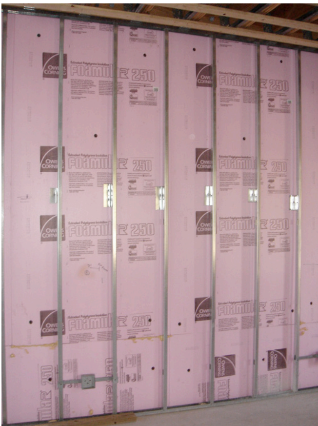
Photograph 3: Vapor Semi-Permeable Rigid Insulation —Note the steel stud interior wall framing is supported by brackets that do not penetrate the foam insulation but are installed over the top of the foam insulation.
