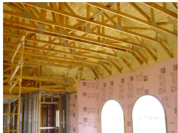
Photograph 5: Unvented Roof —Spray foam insulation applied to the underside of the roof deck bringing the attic and the ductwork inside the conditioned space.
