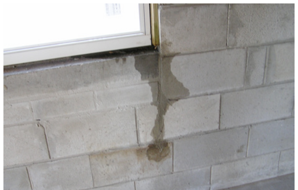
Photograph 4: Leakage Path —Yes, they all really do leak; at the window-to-wall interface and through the window itself.
