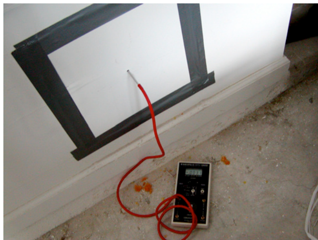
Photograph 7: Pressure Measurement —Return platform goes negative due to return leakage.
