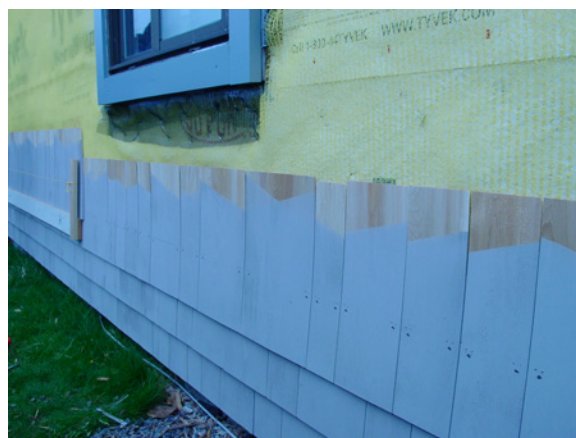
Photograph 4: Cedar Shingles —Back ventilation and drainage of wood shingle cladding installed over OSB covered housewrap – it does not get better than this from a durability perspective.
