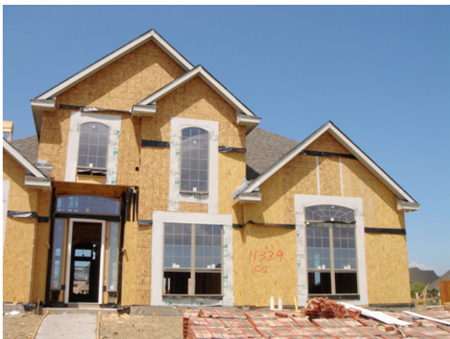
Photograph 1: Ubiquitous Sheathing —A pretty familiar sight – a home completely sheathed with oriented strand board (OSB); “ruling the range...”
