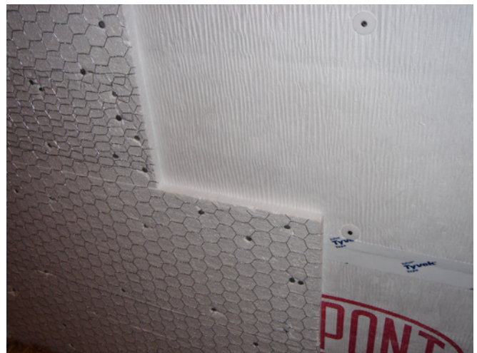
Photograph 9: Water-Managed Claddings —Note the “crinkled” housewrap providing relief of hydrostatic pressure, providing lateral “hygric redistribution” and protection of the OSB (i.e. the de facto “water control layer”). Stucco can be applied directly to the foam, or any other cladding.
