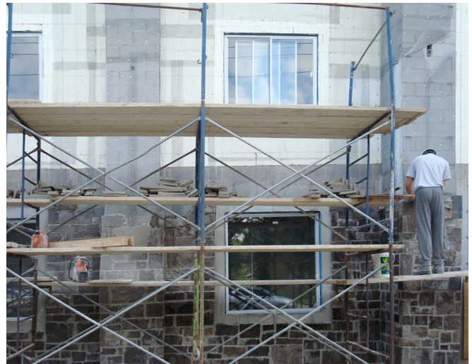
Photograph 5: Manufactured Stone Veneer —Wire mesh set in a cementitious rendering provides the base for an adhered direct applied stone veneer. Think lumpy stucco...
