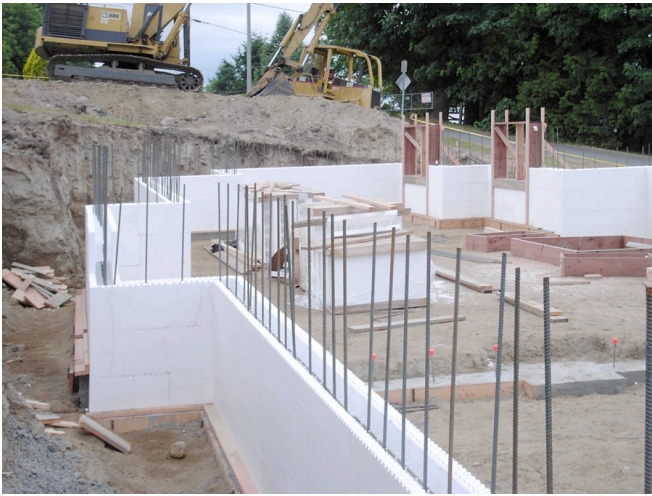
Photograph 3: Foam Building Blocks —Stack 'em up and fill 'em with concrete.
