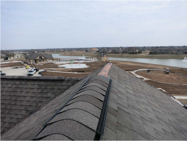
Photograph 10 – Vapor Diffusion Ridge Vent: Standard ridge vent coupled with a vapor open, air tight and water tight membrane covering the slot opening in the roof sheathing at the ridge.
