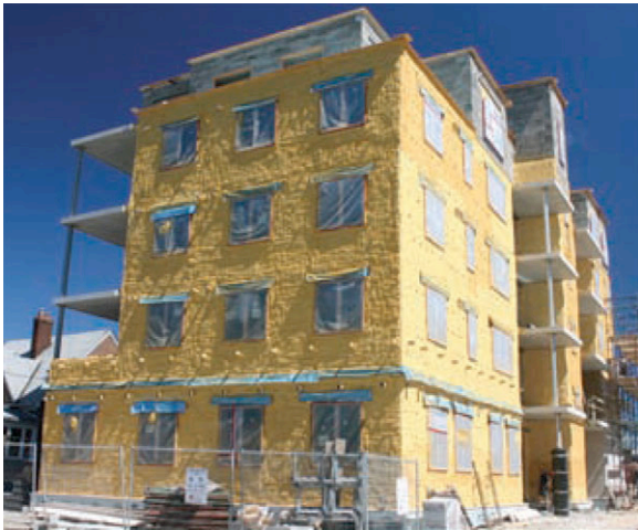
Photograph 2: SPF Applied—Step one.
