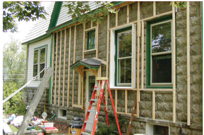
Photograph 13: Wood Frame Off-Set Residential Retrofit —Pretty neat, eh? My friend Peter Yost’s house in Vermont prior to installation of SPF.
