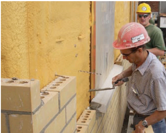
Photograph 3: Brick Installed—Step two.
