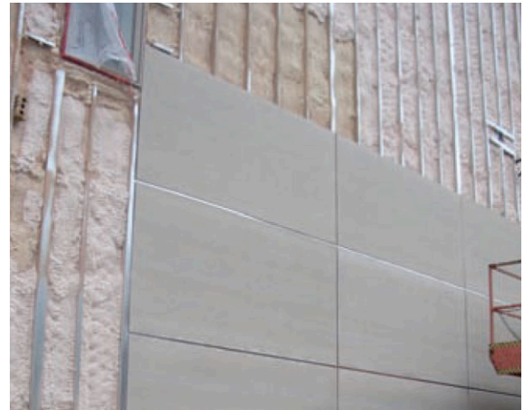
Photograph 5: Vertical channels for panel cladding.
