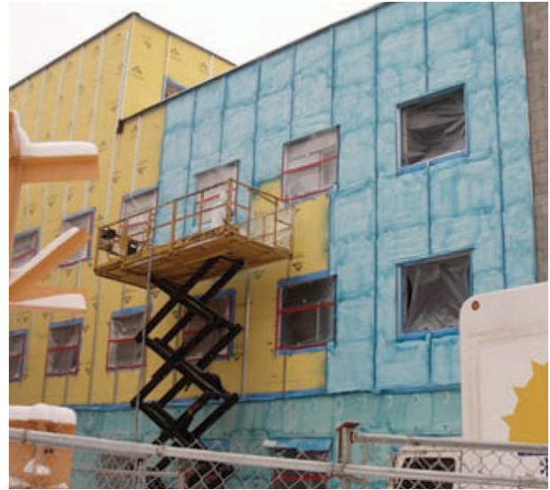
Photograph 9: Z-Bar attachment for panel cladding.
