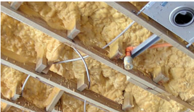
Photograph 11: Air Impermeable Insulation —Spray polyurethane foam is air impermeable. The low density stuff works in the South. The high density stuff works everywhere.
