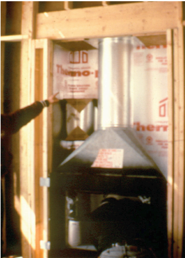
Photograph 8: Draftstopped Fireplace —Pretty easy to get right if you know this is a really big hole. The draftstop makes the fireplace work even better because the fireplace is also warmer. Warm fireplaces draft better. Warm chimneys draft even better.
