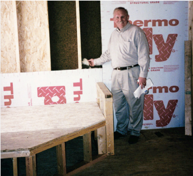
Photograph 5: Effective Draftstopping —Notice the rigid material behind the large soaking tub/whirlpool framing on the exterior wall. Notice the rigid material going up the exterior wall where the shower is going to be. Notice the big smile on the VP of construction for a major, major production home builder in Chicagoland. No comfort complaints for him anymore because there are no big holes.
