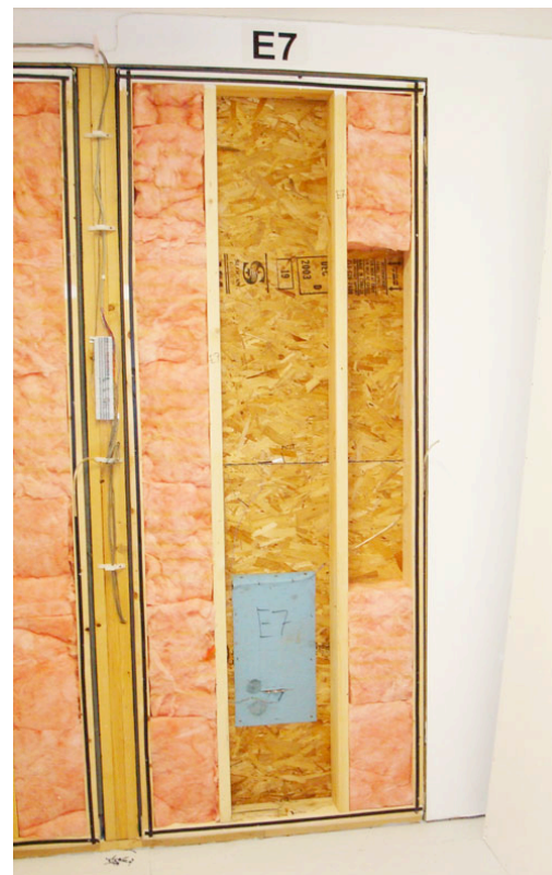
Photograph 8: Interior Wetting Apparatus – Note blue capillary active mat used to distribute water injected into assembly over interior surface of exterior OSB sheathing.
