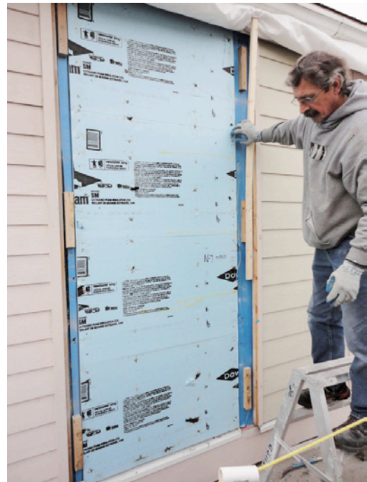
Photograph 7: Stucco over XPS Wall – North elevation deconstruction
