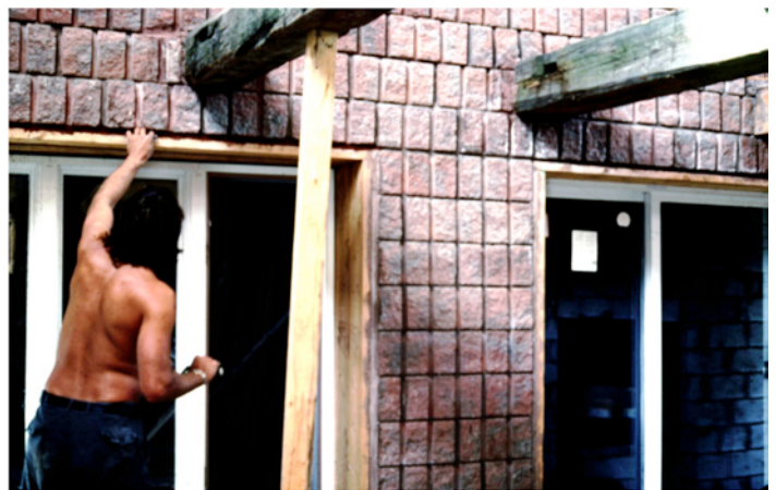
Photograph 3: Interior Finish – Split rib decorative block with exposed structural timbers.
