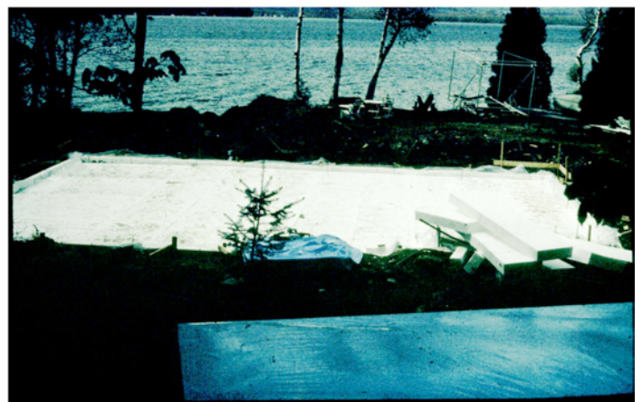
Photograph 8: Slab 2 (above left) – Foam core is embedded into the first layer of concrete as the first layer of concrete is placed. Photograph 9: Slab 3 (above right) – “Foil bathtub” ready for top layer of concrete.
