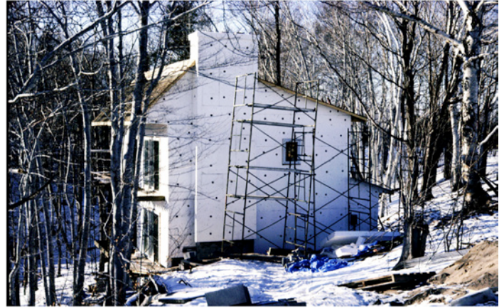
Photograph 4: Energy Trusses (above right) – “High heel” trusses and a R-60 vented attic with an airtight lid. Photograph 5: Exterior Rigid Insulation (above left) – Large plastic washers and mechanically attached 8 inch thick expanded polystyrene (EPS).
