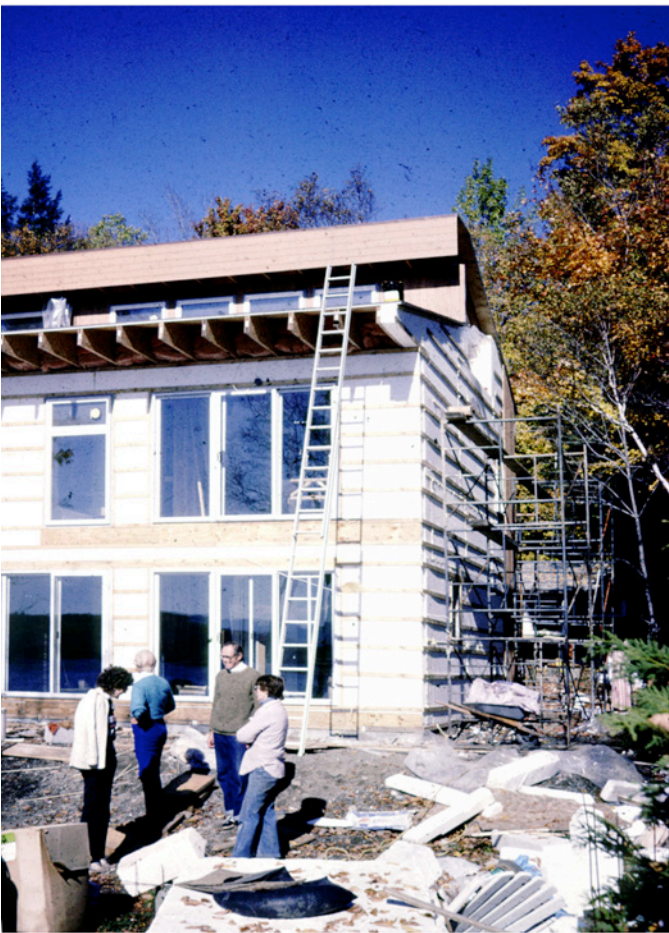
Photograph 11: Frame Structure (top left) - The walls were wood frame sheathed with a new product called oriented stand board (OSB).
