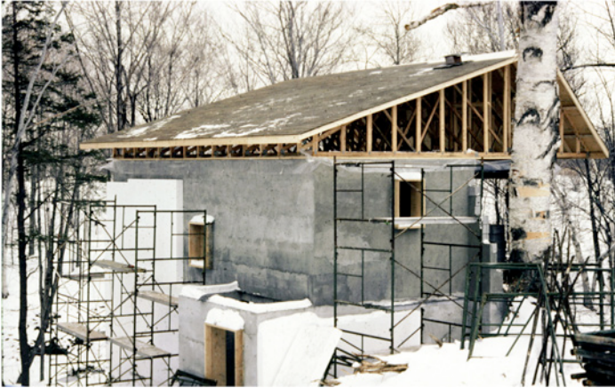
Photograph 4: Energy Trusses (above right) – “High heel” trusses and a R-60 vented attic with an airtight lid. Photograph 5: Exterior Rigid Insulation (above left) – Large plastic washers and mechanically attached 8 inch thick expanded polystyrene (EPS).
