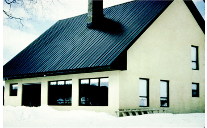
Photograph 1: God’s Country 1979 – Super insulated continuous exterior insulation, triple glazed windows, airtight and ventilated right.
