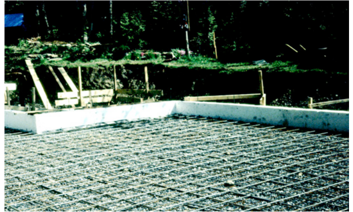
Photograph 6: Go East Young Man (above left) – Wood frame perfect wall in the Eastern Townships outside of Montreal in 1981. Photograph 7: Slab 1 (above right) – Grade prepared for first layer of concrete. Notice the foam form.
