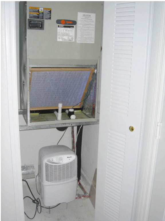
Photograph 6 (above left): Low Tech Dehumidifier —One of those standard-off-the-shelf things that are plumbed such that they drain directly into the condensate drain. Figure 5 (above right): Supply Ventilation System with Intermittent Exhaust —This is a nice system but only works if the outside airflows are low. This system can't work with the new higher Standard 62.2 flow rates.
