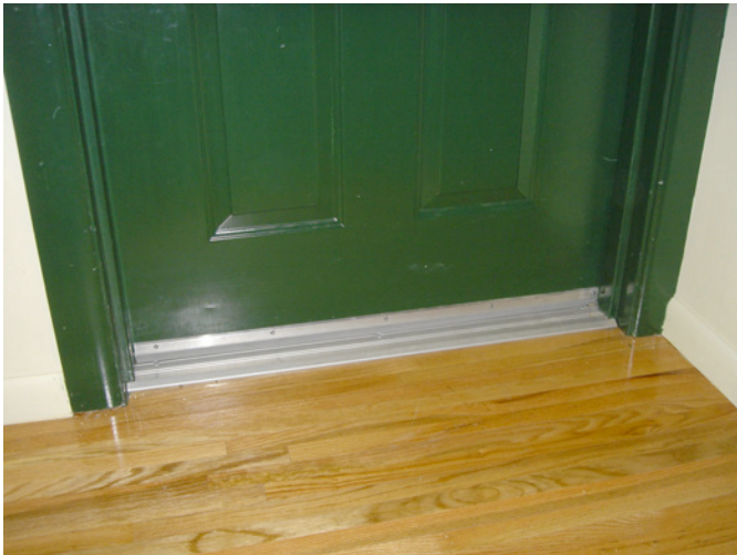
Photograph 4 (above left): Weather-Stripped Door —A beautiful thing if you are worried about fires – an ugly thing if you need make-up air. Photograph 5 (above right): High Tech Big Hole —Good for about 25 cfm, so you need three or four per apartment. They diffuse the incoming air to avoid cold spots and drafts.
