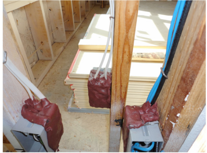
Photograph 2 (above left): More Compartmentalization Air Sealing —Bottom of walls are sealed fabulously well when gypcrete floors are used. Photograph 3 (above right): Airtight Electrical Box —Putty pads are used to seal electrical boxes airtight. Joint compound is used to complete the seal between the electrical box lip and the cut opening in the gypsum board.
