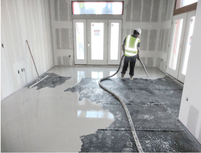
Photograph 2 (above left): More Compartmentalization Air Sealing —Bottom of walls are sealed fabulously well when gypcrete floors are used. Photograph 3 (above right): Airtight Electrical Box —Putty pads are used to seal electrical boxes airtight. Joint compound is used to complete the seal between the electrical box lip and the cut opening in the gypsum board.
