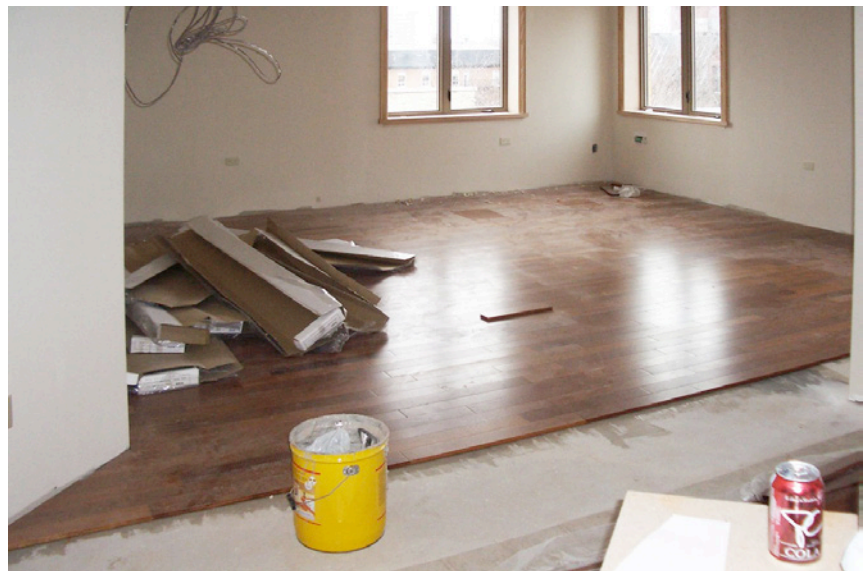
Photograph 5: Glue Down Wood Floor —A decade old and still going strong. Amazing what works if the concrete is dry when the wood goes down and stays dry over time.
