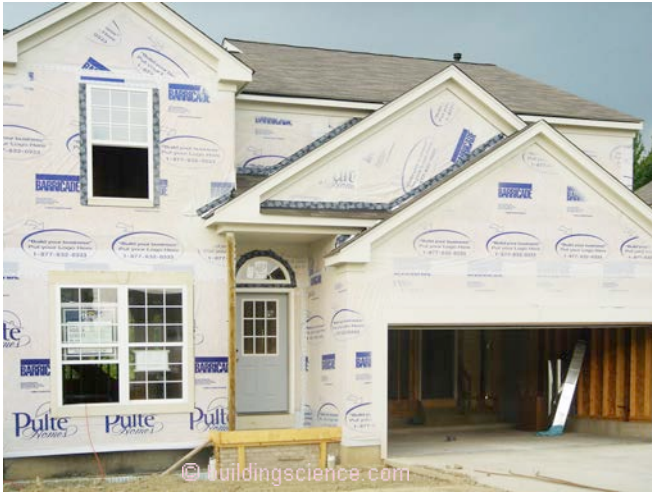
Photograph 6: Air Infiltration Barrier —Classic housewrap rainwater control layer and air control layer. Note the beautiful job of flashing integration with the housewrap. The outside is the right place for air control.
