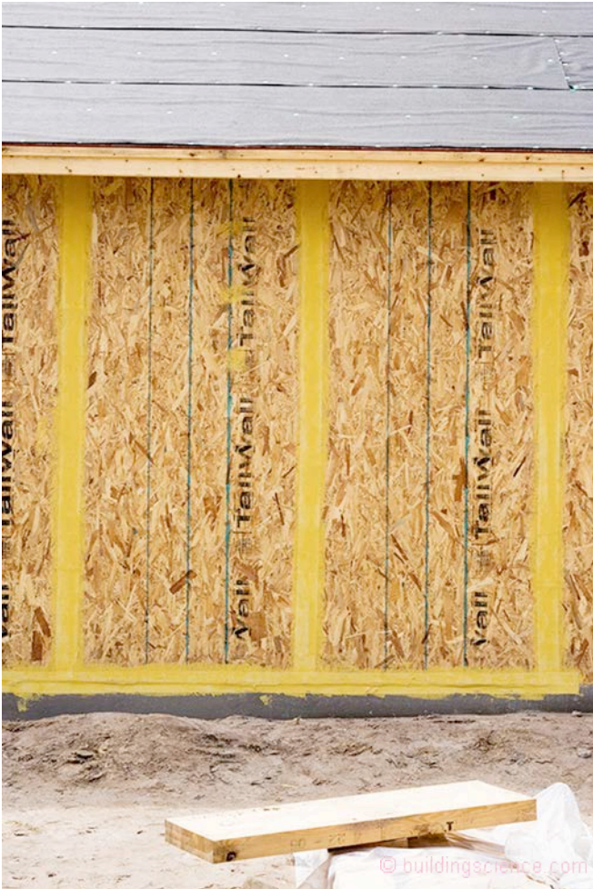
Photograph 16: Fluid Applied Joint System —Replacing tapes with fluid applied joint systems is now possible.
