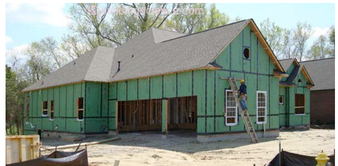
Photograph 14: Sheathing Water and Air Control Layer —The sheathing in this system is pre-coated with a water control layer. Tape is used provide water control and air control layer continuity.
