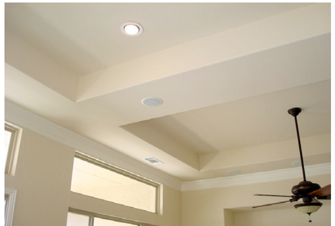
Photograph 2: Dropped Ceiling “Look” – Not everyone likes the look of dropped ceilings.
