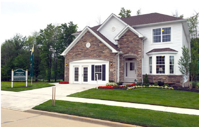
Photograph 7: Test House – One of several standard production houses located in various climate zones used to test buried ductwork configurations.
