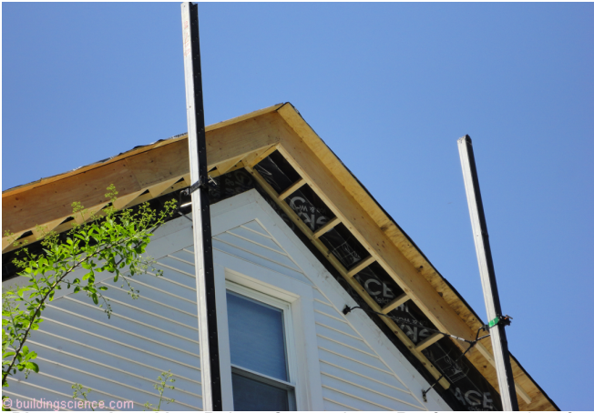
Photograph 5: More Robust Connections - Roof eaves and roof rakes experience the highest positive and negative air pressures. The structural connections connecting the roof deck layers to the wall assemblies need to be “robust”.
