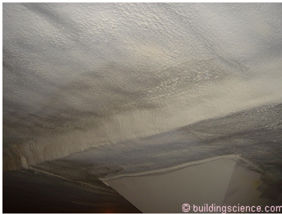
Photograph 2: Closed Cell Spray Polyurethane Foam – This approach works in all climate zones.
