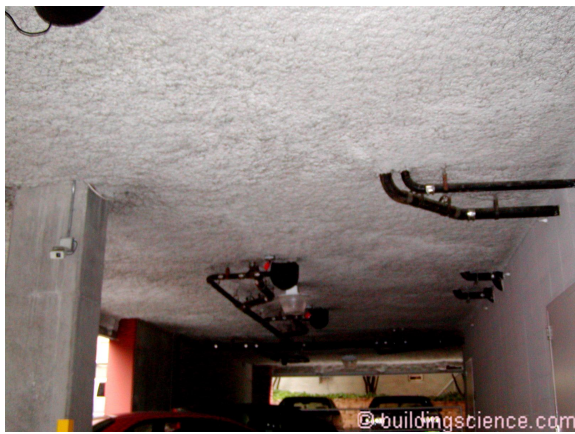
Photograph 3: Closed Cell Spray Polyurethane Foam – The spray foam requires a spray applied cementitious or fiber fireproofing layer installed over it.
