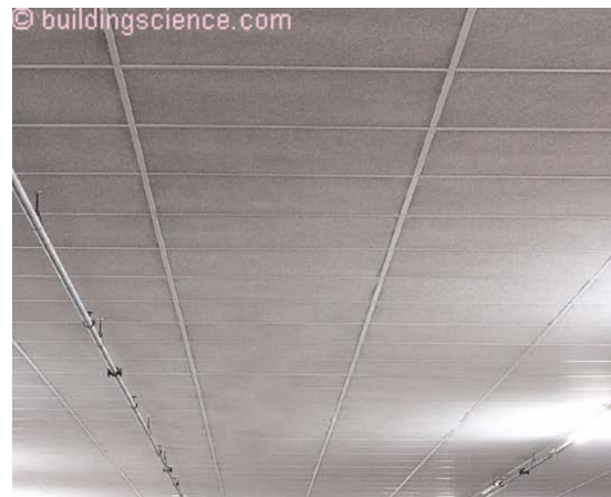
Photograph 4: Lay-In Ceiling Tiles – Insulate the top of the lay-in ceiling tiles with fiberglass or mineral wool batt insulation.
