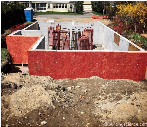
Photograph 5: Exterior Rigid Insulation – High density fiberglass rigid insulation which provides exterior drainage and control of hydrostatic pressure.
