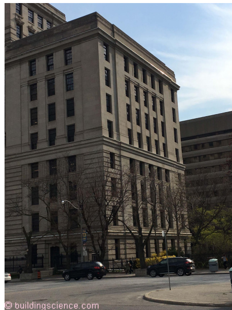
Photograph 9: Canada Life Building in Toronto - We messed up the building during the depression years...but fixed it with retrofitted drip edges.
