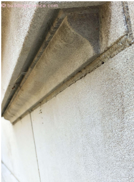
Photograph 2: Kerf - Kerf cut into the underside of the stone sill in Washington, DC a hundred years ago.
