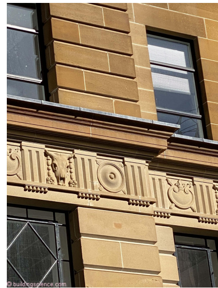
Photograph 11: New Zealand Retrofit Drip Edges – Wellington, New Zealand...they drive on the wrong side of the road...but they do know buildings...
