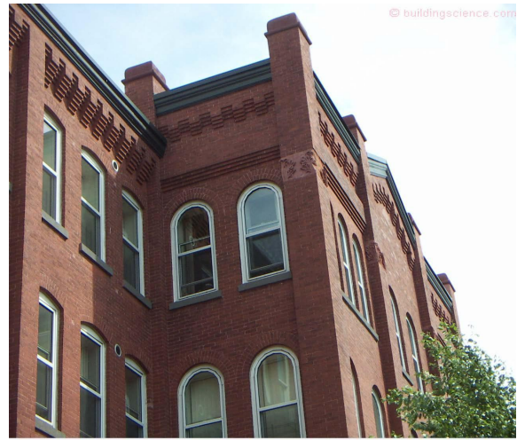
Photograph 13: Parapet Drip Edge - Retrofitted “reversible” parapet coping drips.
