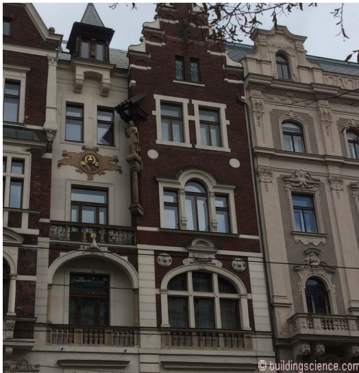
Photograph 12: Czech Republic – Lots of drip edges...no risk of freeze-thaw...
