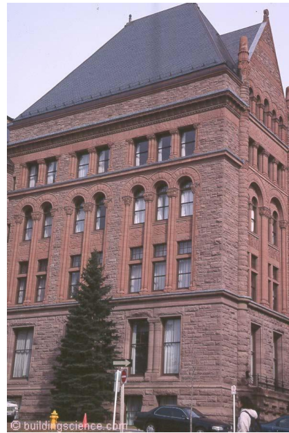
Photograph 8: Ontario Legislature Assembly - We got it wrong in Toronto on our Legislature Assembly a hundred years later and had to add drip edges.
