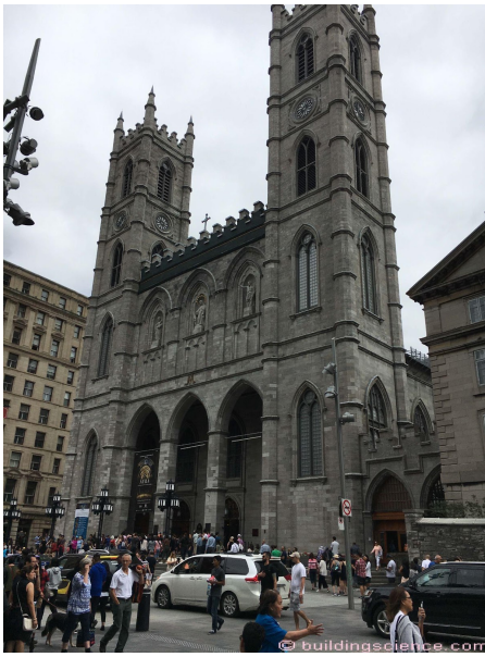
Photograph 6: Notre-Dame Basilica in Montreal - Look closely at the horizontal “bands”....they were supposed to act as “drip edges”...
