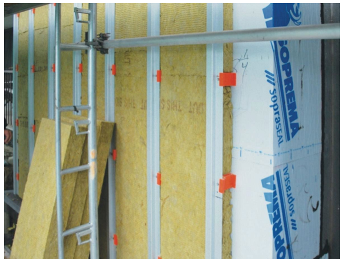
Photograph 1: Non-Thermally Conductive Fiberglass “Clip”
