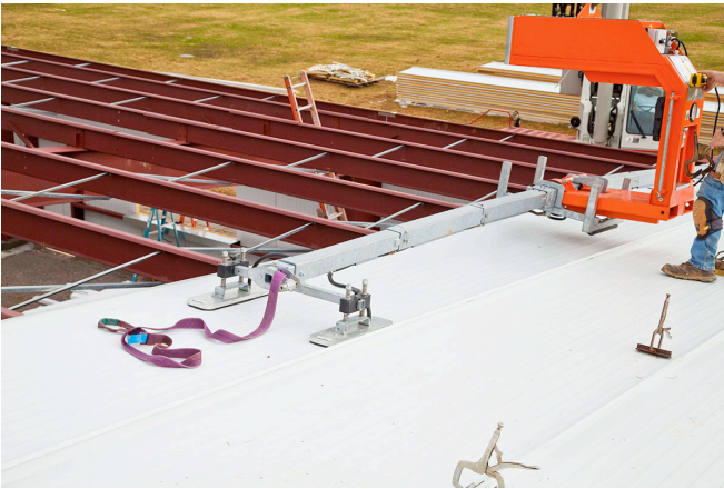
Photograph 5: Insulated Metal Roof Panel —Positioning the roof panel during installation.
