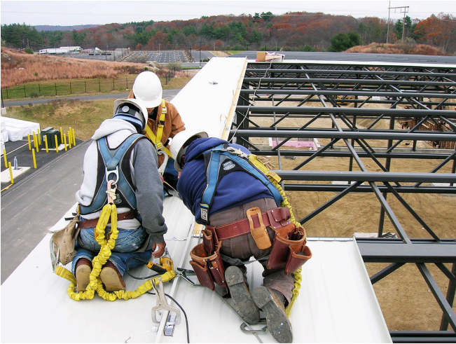
Photograph 4: Insulated Metal Roof Panel —Installation of roof panels “crimping” the “standing seams”.
