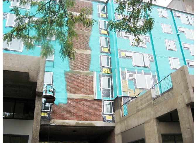
Photograph 6: Retrofit Metal Panel —With retrofit approaches it is common to apply a fluid water and air control layer directly to the masonry. Note the sheet membrane transition between the field of the wall and the replacement glazing system.
