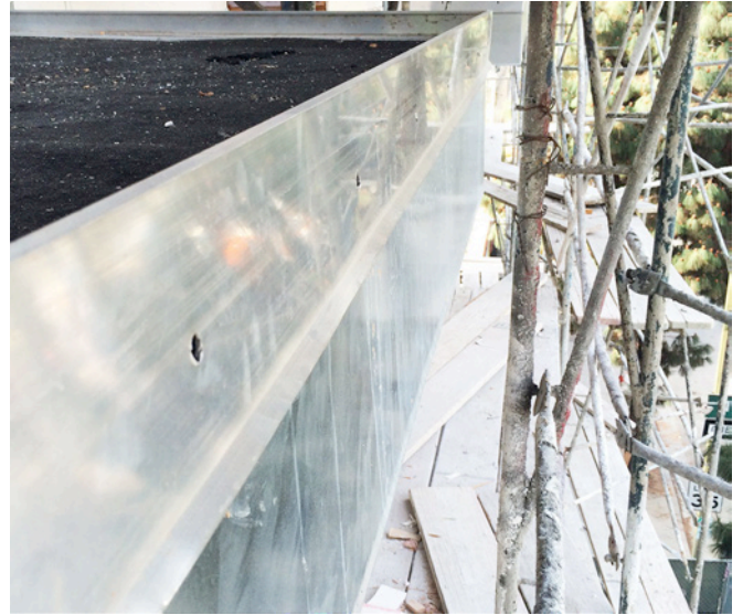
Photograph 9: Two Drip Edges —The upper drip edge sheds water flowing over the edge of the concrete topping. The lower drip edge sheds water from the drainage mat gap on the top of the waterproofing membrane under the concrete topping. This two-stage drip edge approach is recommended to deal with any minerals carried in solution in drain water exiting the drainage mat gap.
