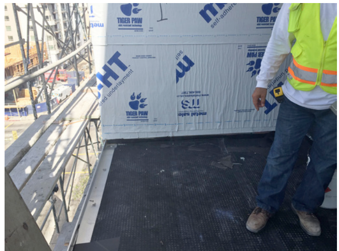
Photograph 7: Drip Edge and Drainage Matt —The water resistive barrier (WRB) is lapped over the membrane waterproofing. A drainage mat is in place as is the drip edge at the balcony edge.
