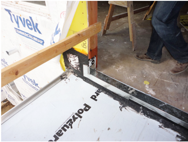
Photograph 4: Membrane Waterproofing —Additional metal flashing is installed over the waterproofing that is stripped into the pan flashed balcony door opening. This additional metal flashing protects the membrane waterproofing at the door opening.
