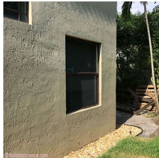
Photograph 1: Pea Gravel – Crushed Stone Perimeter Pest Resistant Ground Break
