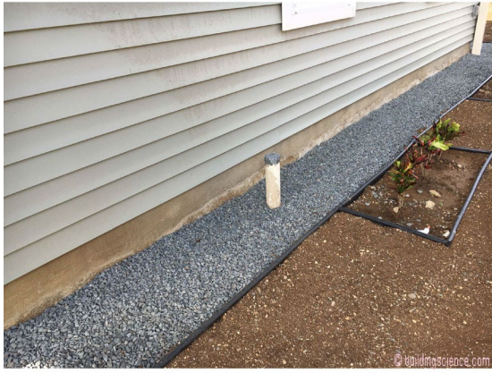
Photograph 2: Pea Gravel – Crushed Stone Perimeter Pest Resistant Ground Break
