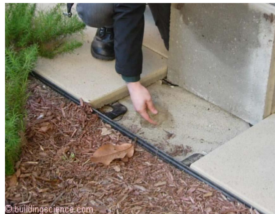
Photograph 5: Concrete Paver Perimeter Pest Resistant Ground Break (photograph courtesy of the San Francisco Department of the Environment - Pest Prevention by Design)
