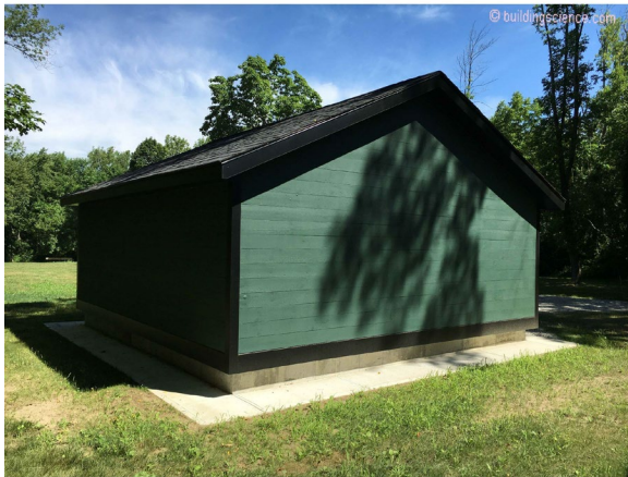
Photograph 3: Concrete Skirt Perimeter Pest Resistant Ground Break
