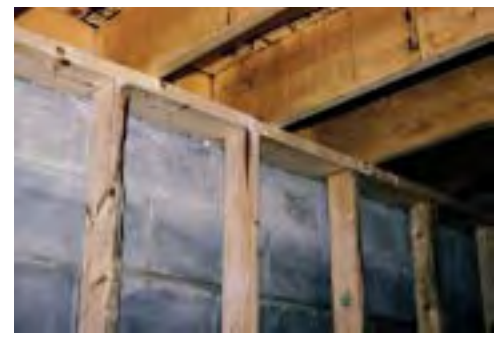
Photograph 1 Interior stud framing located at basement perimeter
