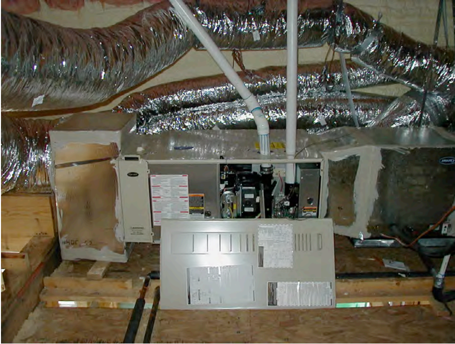
Figure A-6a Photograph of air handler unit of 2-stage compressor with ECM fan and Thermidistat system
