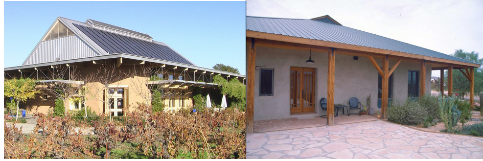
Photographs 4 and 5: Generous roof overhangs provide shading and shelter for these strawbale buildings
