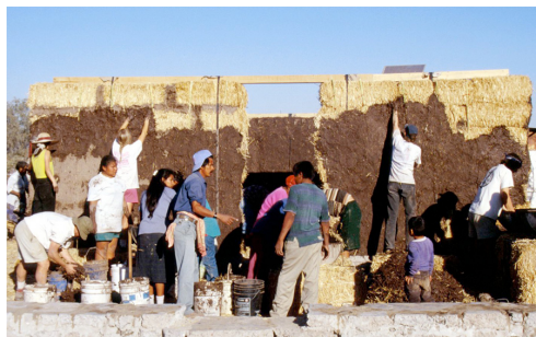
Photographs 1 and 2: Strawbale walls can be built with locally available materials and community labor (left) and are often chosen for their sculpted, massive aesthetics (right).
