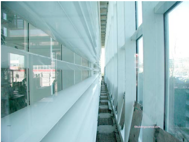
Photograph 2: Mind the Gap —More Hooker Chemical Company building double façade. Not a heck of a lot more to needs to be said here. The population of a small village could live in this space.
