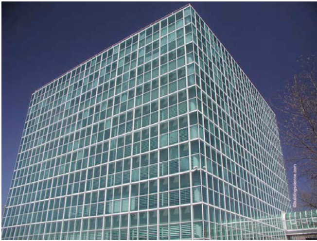
Photograph 1: Hooker Chemical Company —The folks that brought us the Love Canal also brought us the first double façade building in the United States in the 1970's.
