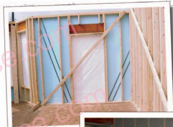
Continuous rigid insulation for thermal break
