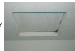
Attic access hatch in the master bedroom closet
