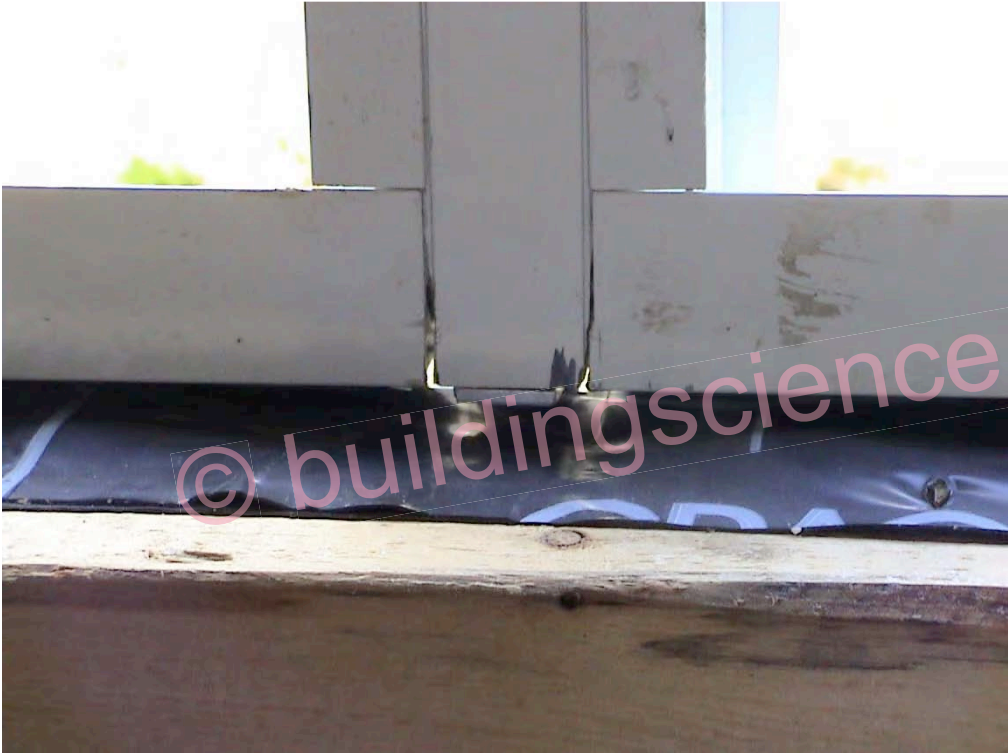
Photograph 26: Mulled Window Unit Leakage Paths
