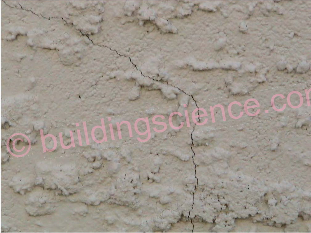
Photograph 61: Water Entry Associated With Typical Crack In Stucco Rendering
