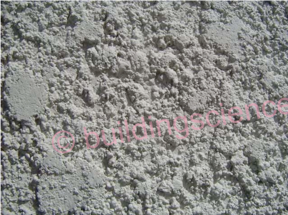
Photograph 66: Paint Coating Over Rough Surface
