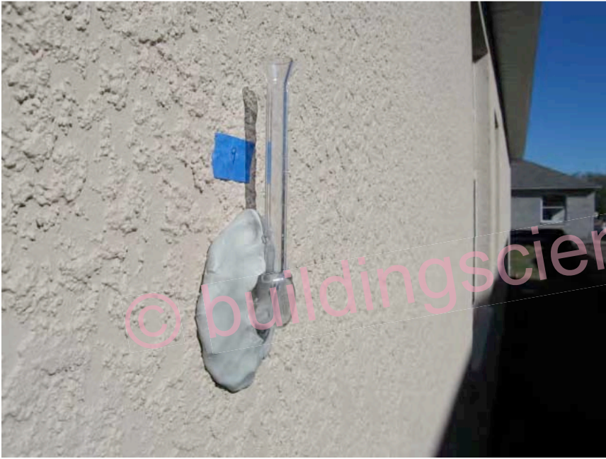
Photograph 43: Rilem Tube Hydrostatic Head Test
