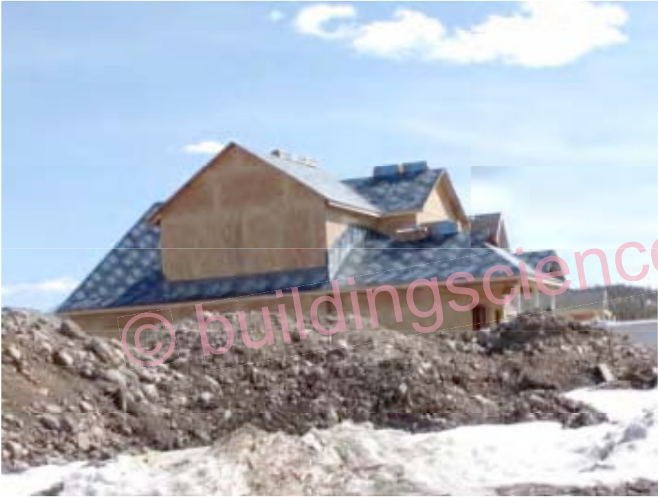
Photograph 72: Direct Applied Self Adhering Membrane
