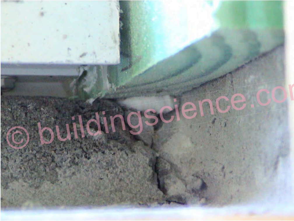
Photograph 26: Mulled Window Unit Leakage Paths
