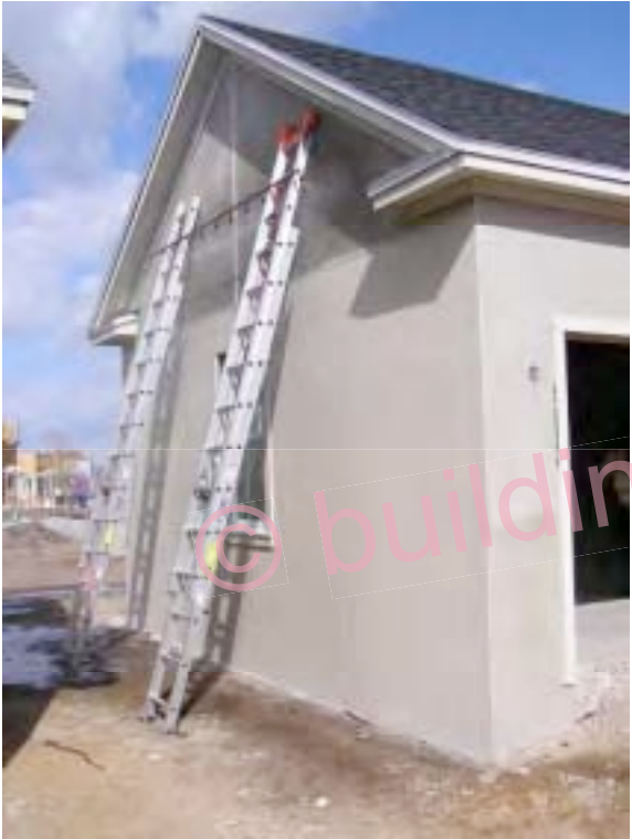
Photograph 59: Water Testing – Control Joints
