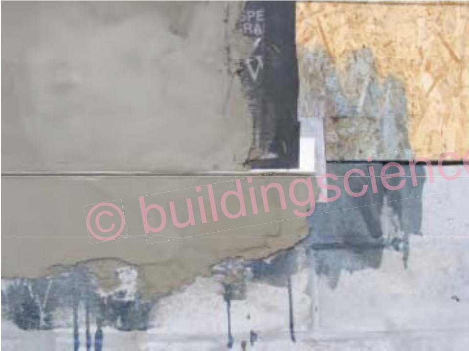
Photograph 22: Stucco Rendering Applied At Draining Control Joint
