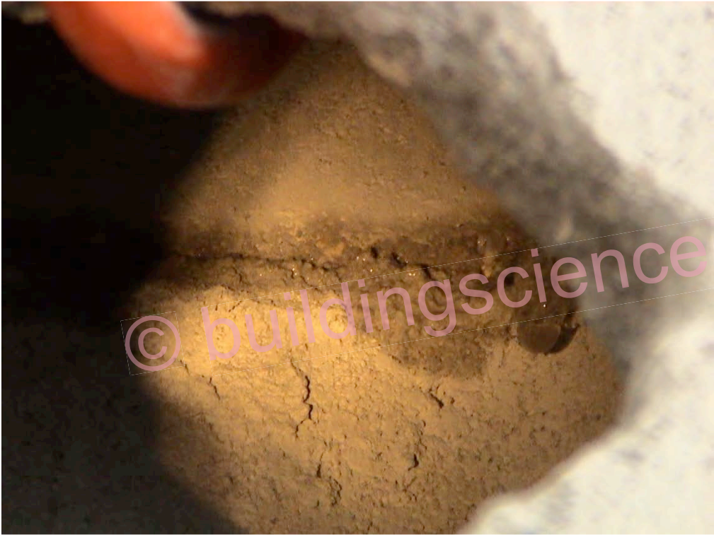
Photograph 61: Water Entry Associated With Typical Crack In Stucco Rendering
