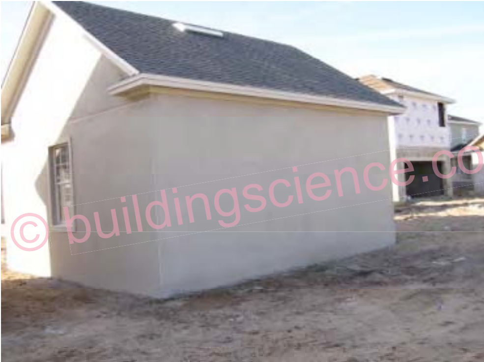
Photograph 53: Painted Stucco Rendering Test Wall
