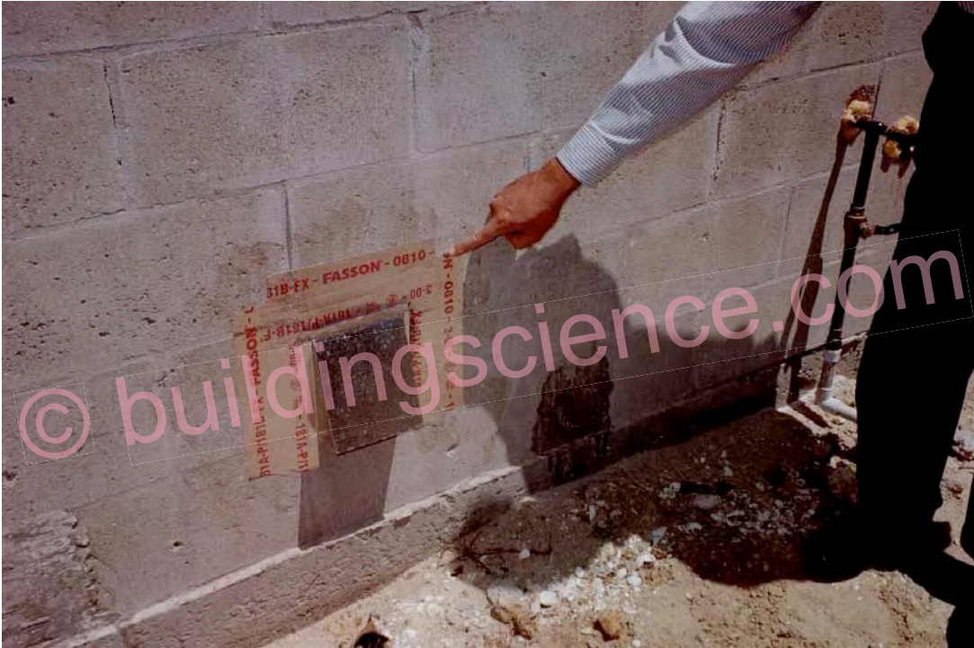
Photograph 36: Flashed Electrical Box
