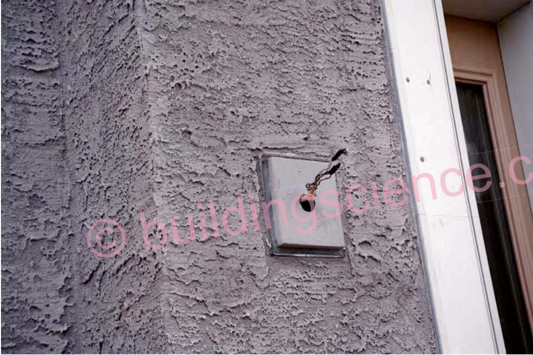
Photograph 36: Flashed Electrical Box
