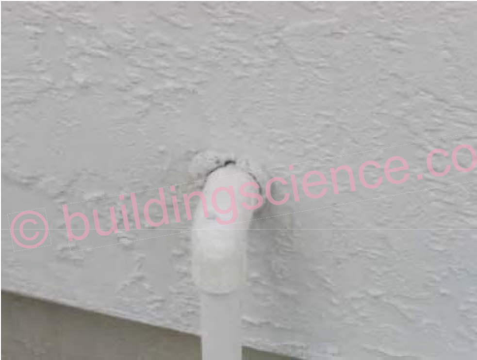
Photograph 34: Dryer Vent Opening
