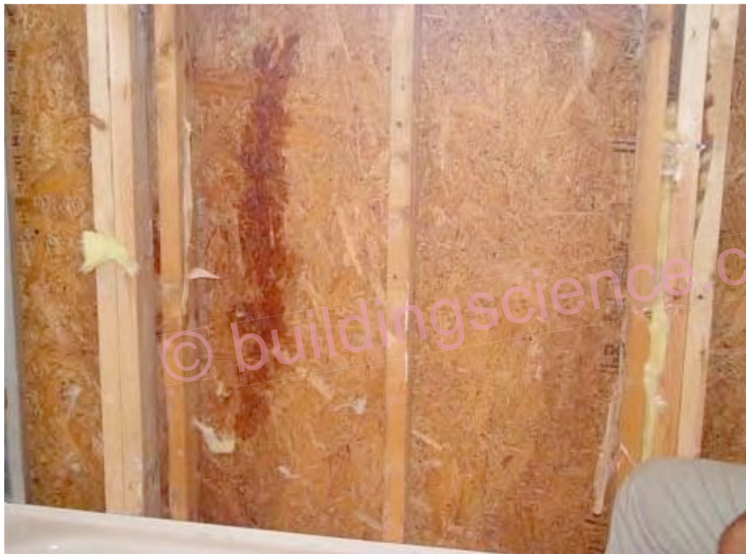
Photograph 2: Rainwater Entry into Second Floor Frame Assembly
