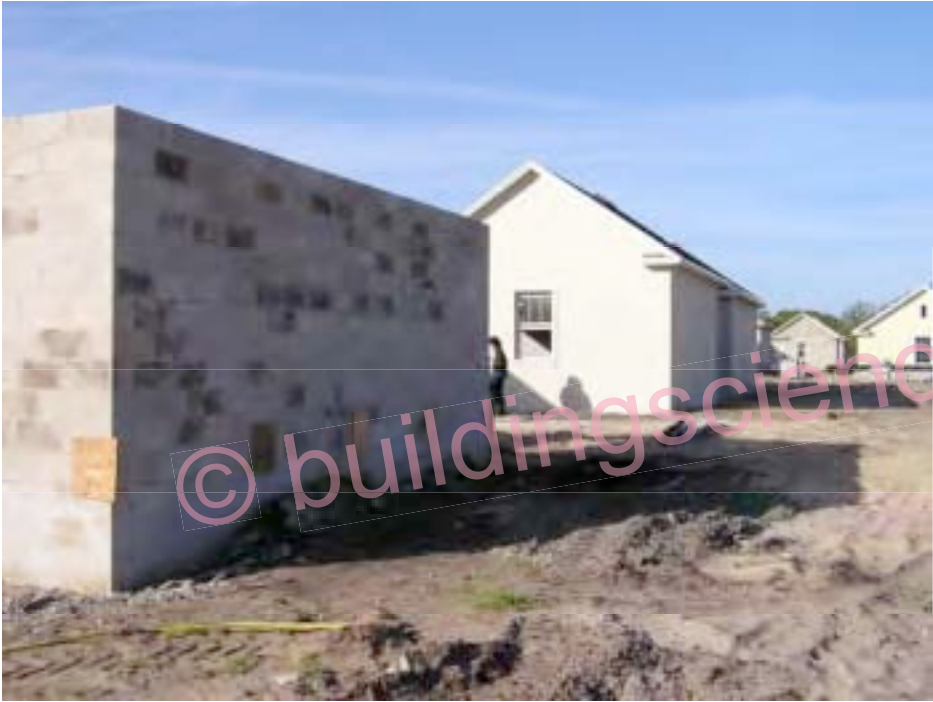
Photograph 51: Garages Used As Test Walls – Varying Configurations
