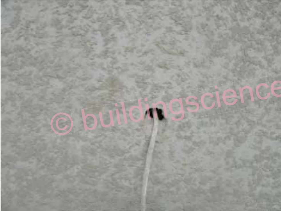
Photograph 32: Typical Maintenance Intensive Service Opening
