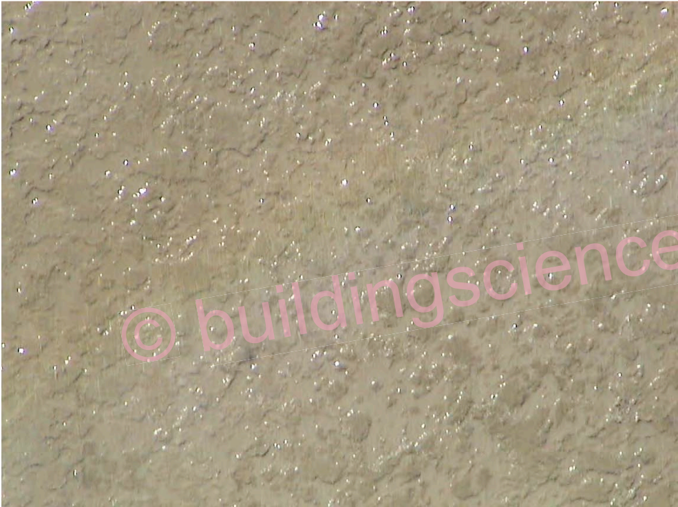
Photograph 70: Fiber Reinforced Stucco Rendering to Control Cracking
