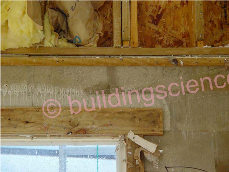
Photograph 17: Water Entry Between Floors
