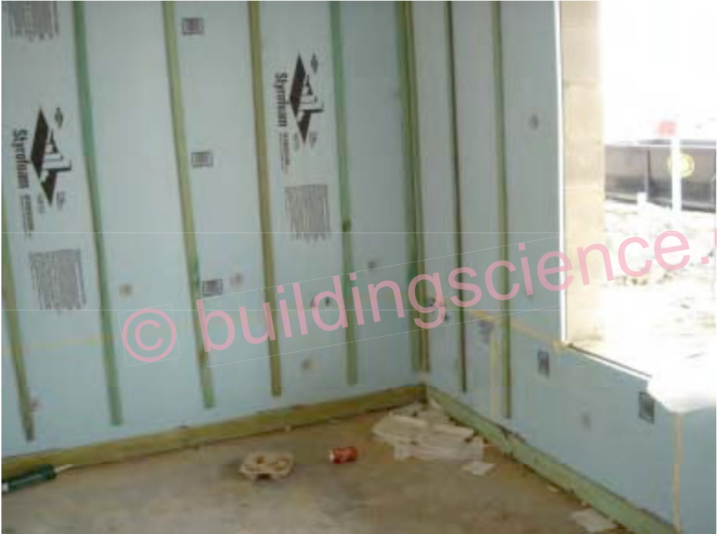
Photograph 64: Rigid Foam Interior Lining Protecting Interior Surfaces
