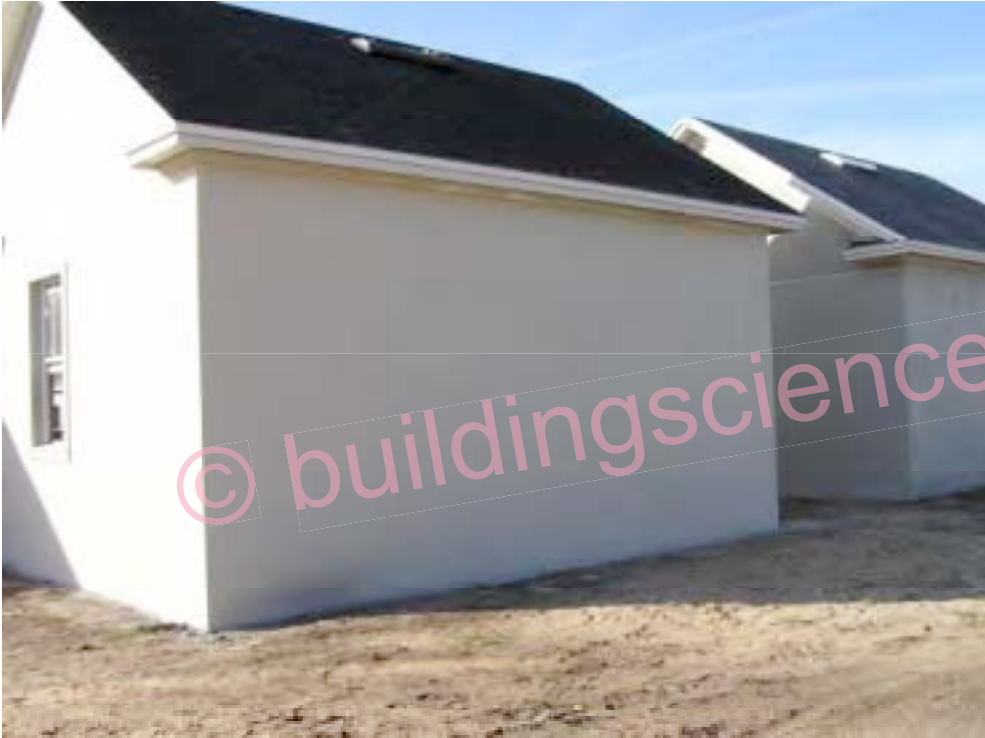
Photograph 53: Painted Stucco Rendering Test Wall
