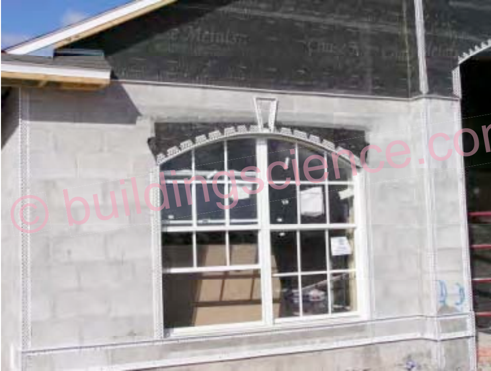
Photograph 24: Window Corner Leakage
