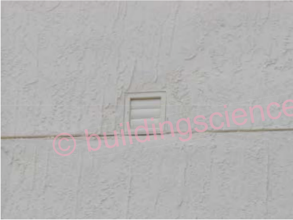
Photograph 34: Dryer Vent Opening
