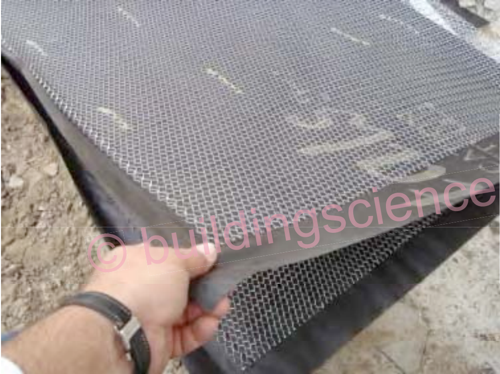
Photograph 12: Paper Backed Lath As A Bond Break
