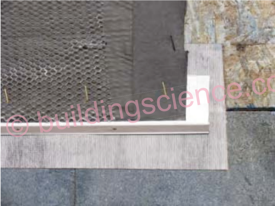
Photograph 22: Stucco Rendering Applied At Draining Control Joint
