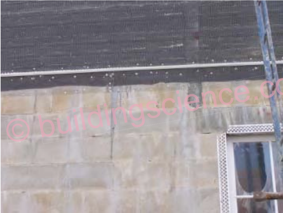
Photograph 17: Water Entry Between Floors
