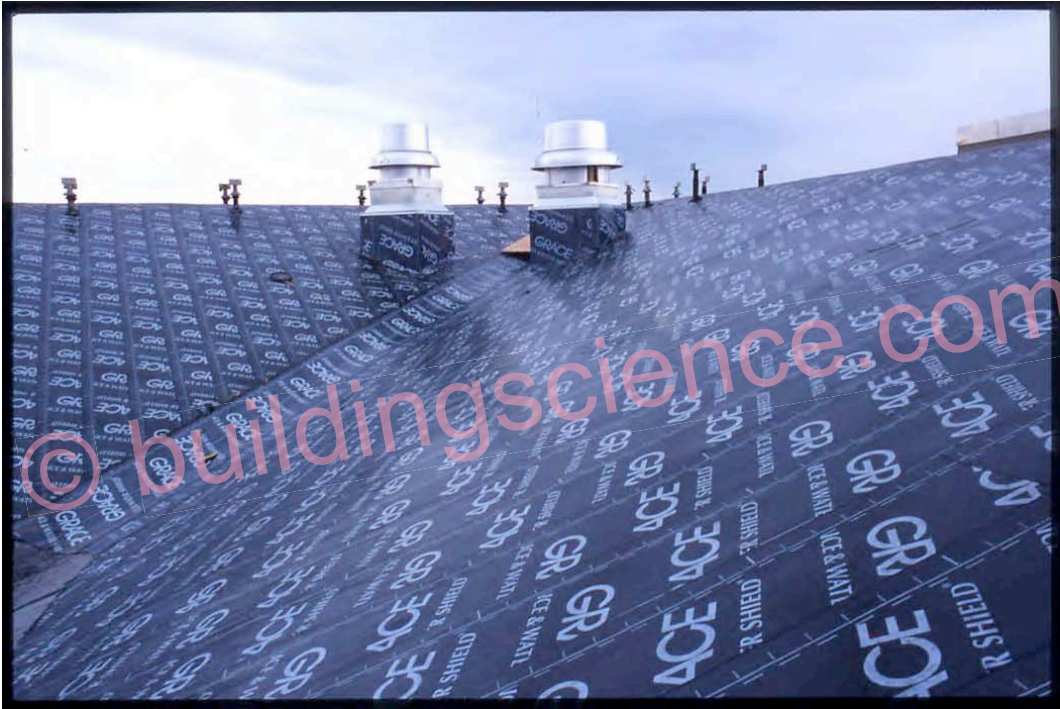
Photograph 73: Large Institutional Roof – Direct Applied Self Adhering Membrane
