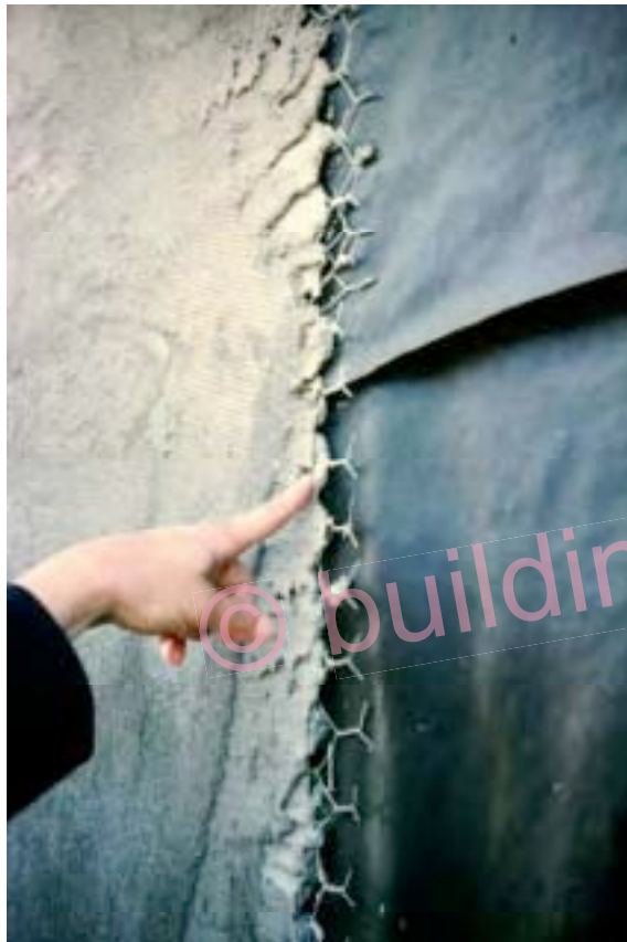
Photograph 3: Stucco Rendering Bonding to Building Paper
