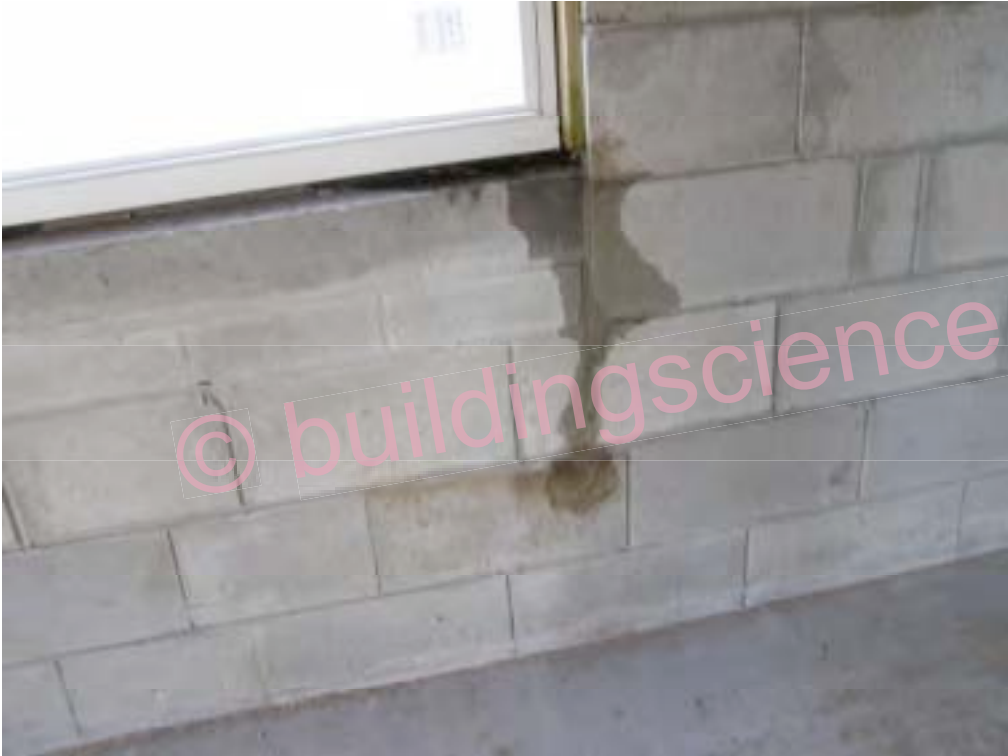
Photograph 24: Window Corner Leakage
