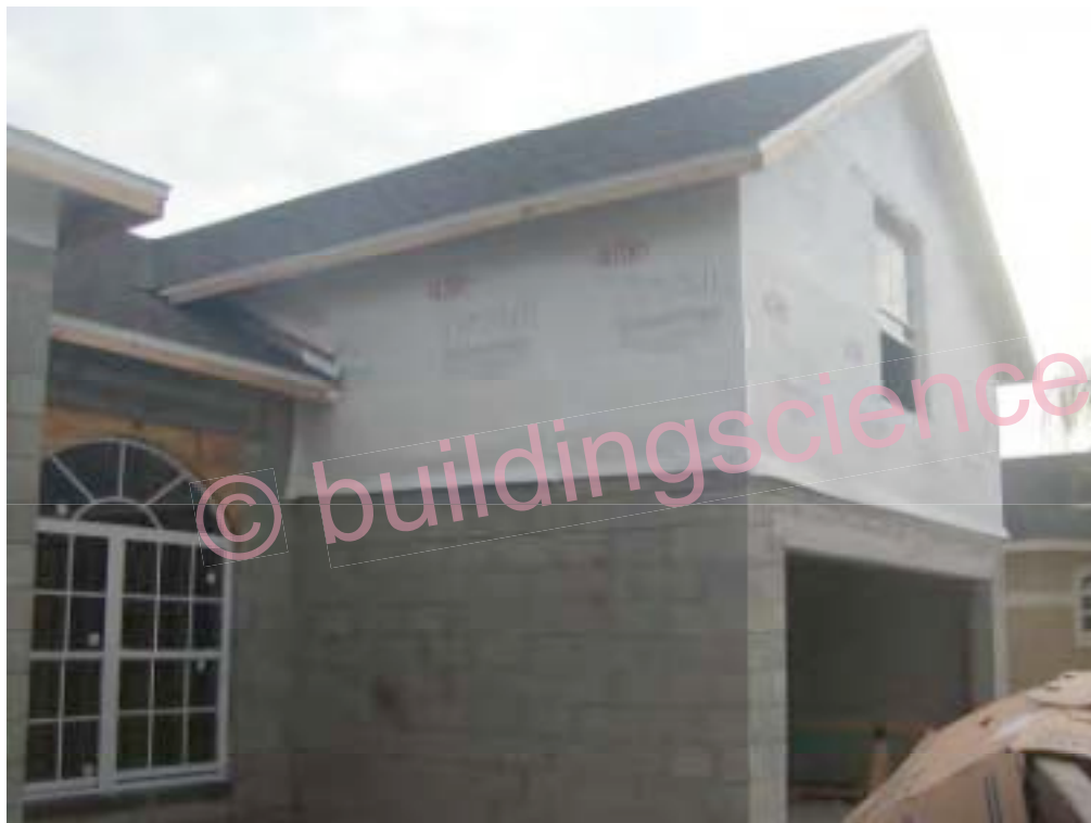
Photograph 13: Enhanced Drainage With A Profiled Plastic Housewrap
