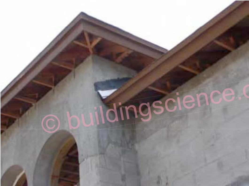
Photograph 40: Mastic Adhered Kick Out Flashing On Mass Assembly
