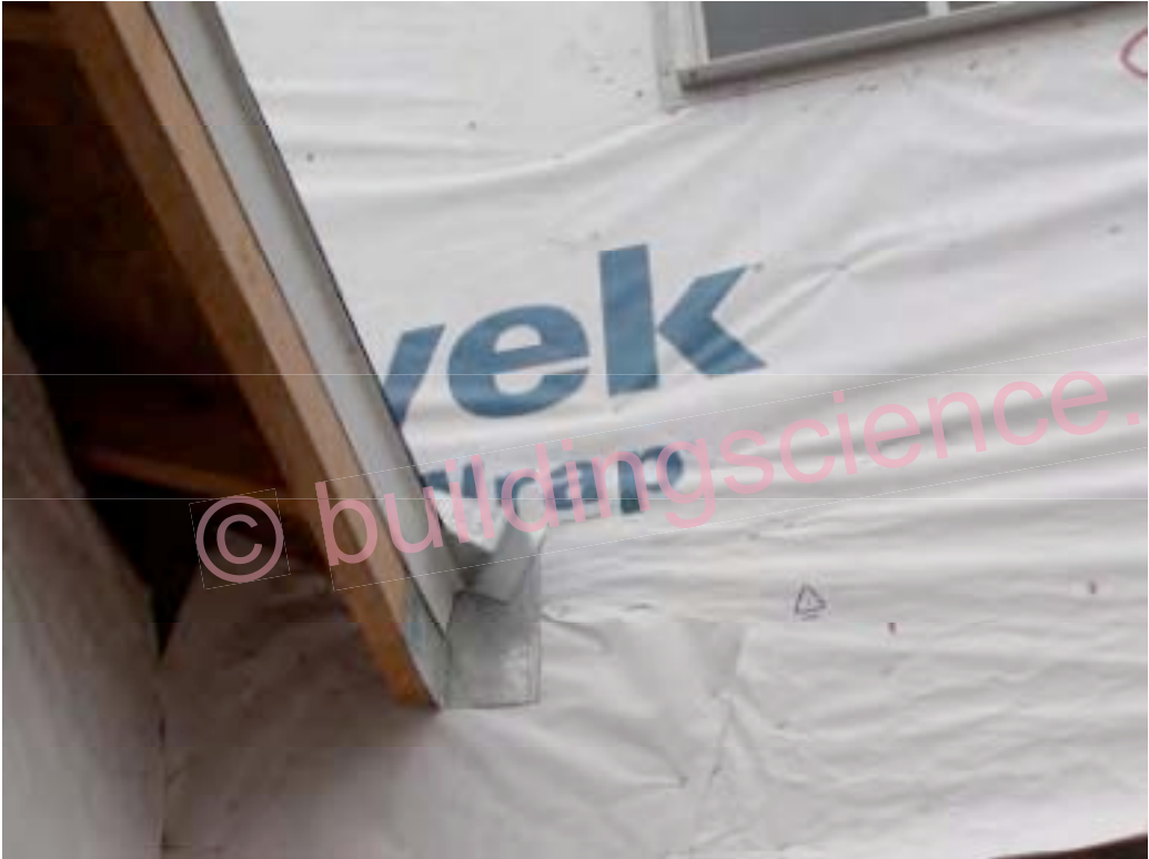
Photograph 38: Recommended KickOut Flashing Detail
