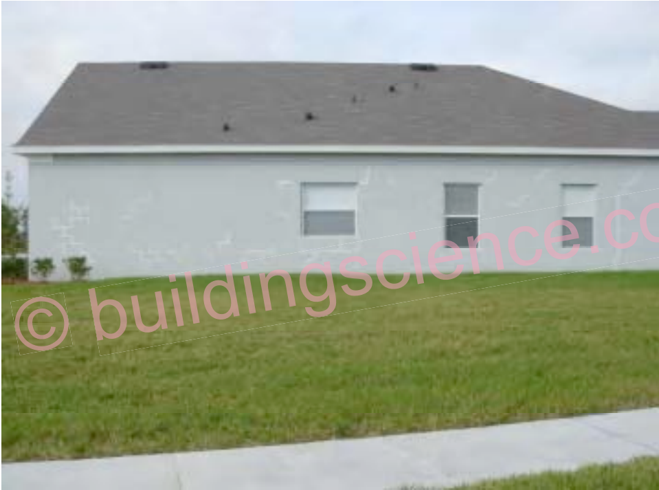
Photograph 70: Fiber Reinforced Stucco Rendering to Control Cracking
