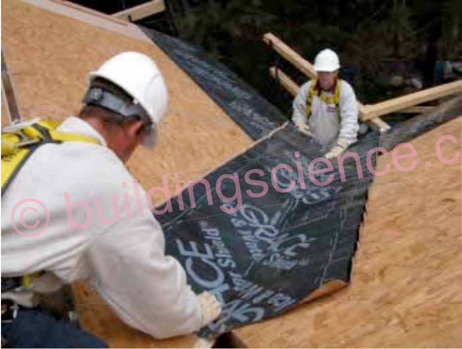
Photograph 71: Self Adhering Membrane
