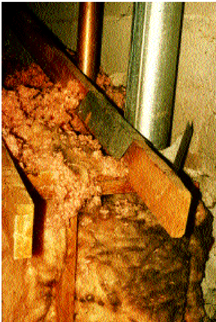
Fiberglass insulation is a filter, not an air-barrier. Note the dark markings (filtered dust) in the material.
