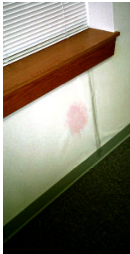
Photo A. Typical mold “pink spot” created when organism releases digestive enzymes that react with plasticizers in the wall.
