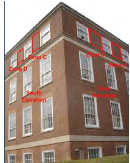
Picture 1. Exterior south-east corner. All wall mock-up zones shown, zones A/B (east elevation), zones C/D (south Elevation).
