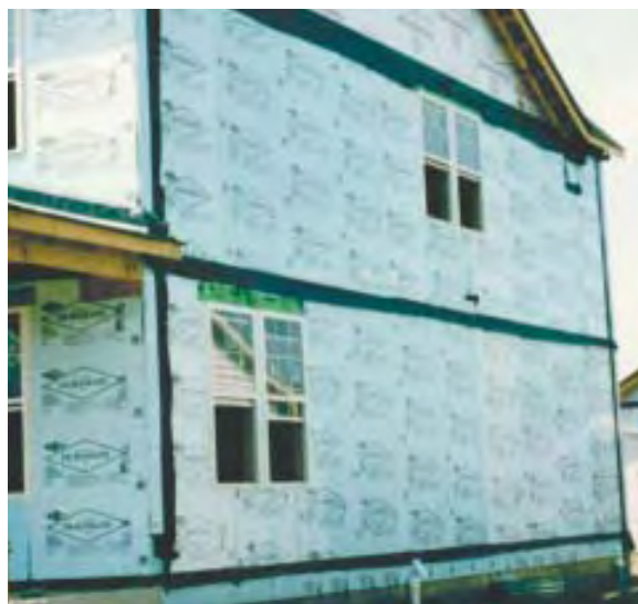
Figure 7. Extruded polystyrene or foil-faced polyethylene can be an effective drainage plane material. Joints in the foam can be taped with red Tyvek tape (top). To reduce reliance on tape or sealant, the author likes to apply the foam with shiplap joints at the vertical seams and a black poly strip as a Z-flashing at horizontal joints (right).
