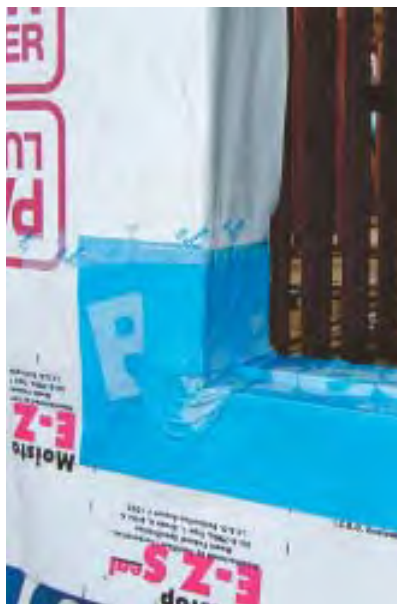
Figure 8. Sealing window flanges to the housewrap (far left) is a common practice, but it does not protect against the predictable leakage within the window assembly itself. Only a pan flashing that dumps on top of the drainage plane will effectively keep water out of the wall. Peel-and-stick membrane applied over the top of the building paper and wrapping the sides and bottom of the rough opening (left) accomplishes the task. A preformed metal pan flashing with soldered joints (below) also works. The author highly recommends Tyvek FlexWrap for pan flashings, whether the drainage plane is housewrap or rigid foam (below left).
