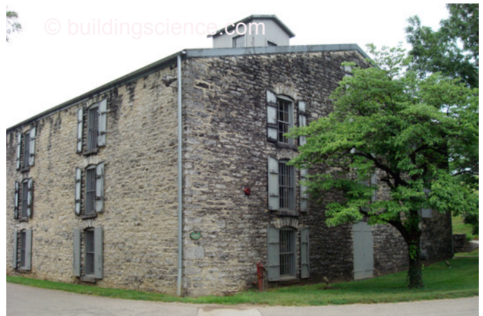
Photograph 9: “Angels Share” —Legend has it that the mold growth on the exterior of old bourbon warehouses is due to the evaporation of alcohol from the barrels and the subsequent diffusion of this alcohol through the walls providing nutrients to support mold growth. The “missing” alcohol from the barrels is called the “angels share”. Of course sometimes mold is just mold (yes, sometimes a cigar is just a cigar...).
