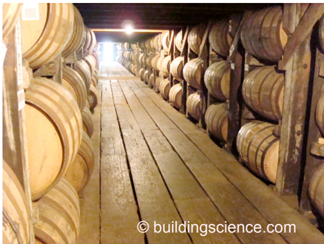
Photograph 4: A Beautiful Sight —Notice that the barrels are stored in a manner that allows air circulation. Warehouses don’t have “floors” in the typical sense. They have “catwalks” between stacks of barrels that are both cross-ventilated and stack (air flow from down low to up high) ventilated.
