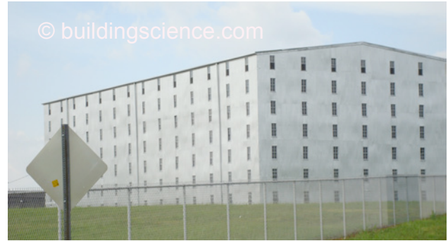
Photograph 7: Low Thermal Resistance/High Reflectivity Warehouse —“Shiny” metal cladding, “shiny” metal roof, open wood frame, no thermal insulation. The thermal control is radiation and ventilation based. High solar reflectivity of the wall and roof “knocks” the peaks off the high temperature extremes – rejecting solar radiation in the summer. Low emissivity of the wall and roof “fills” the valleys in the low temperature extremes – reducing radiation heat loss during cold weather. Cross ventilation and stack ventilation further moderate the temperature. Translation, building does not get as hot as it could in the summer and as cold as it could in the winter.
