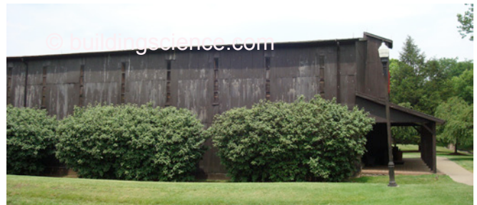
Photograph 8: Low Thermal Resistance/Low Reflectivity Warehouse —Dark (painted) metal cladding, dark metal roof, open wood frame, no thermal insulation. The warehouse is deliberately designed to get hot in the summer and cold in the winter. The roof and wall have high solar absorption gaining heat in the summer. The roof and the wall have high emissivity – increasing radiation heat loss during cold weather. This is the opposite of the approach taken for Low E window glazing – this is a “High E wall and roof”.
