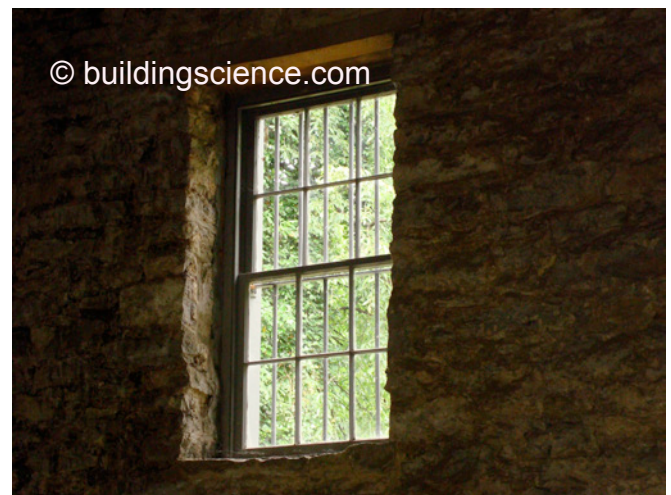
Photograph 6: High Thermal Resistance and High Mass Wall —Not too shabby for a bunch of Cohee’s – I bet around R-5 – with a huge hygric buffer to boot (“hygric buffer” is consultant babble speak for moisture absorption, moisture storage, and moisture desorption).
