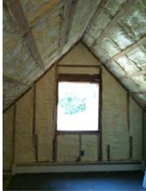
Closed cell spray foam in roof and walls
