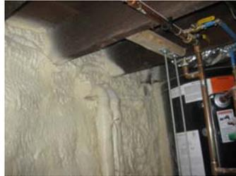
Basement wall insulation before application of ignition barrier paint
