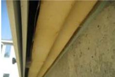
*Polyiso exterior insulating sheathing with housewrap drainage plane and turring*
