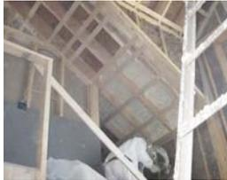
Closed-cell spray foam at roof deck
