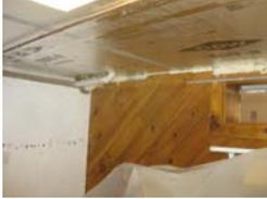
*Foil-faced rigid insulation at basement ceiling*
