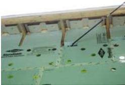
*Exterior sheathing sealed to baffles*
