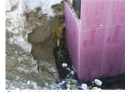
*Exterior insulating sheathing and perimeter drain*
