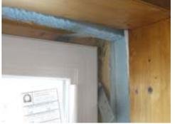
*Window installation from interior before air sealing with foam around window*
