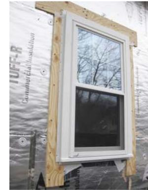
Flanges attached to window strapping
