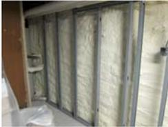
*Metal stud wall over closed cell spray foam*
