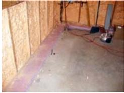
*Thermal break under existing wood stud wall*
