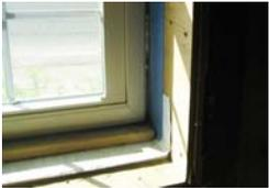
Housewrap and flashing extends into the window box sealed with caulking
