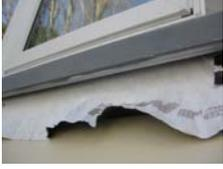
*Window plan flashing extends over cladding*
