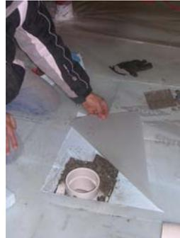
Basement slab system with radon vent
