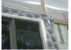
*“Outie” window attached to strapping over rigid insulation*
