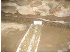
*Interior sub-slab drainage*
