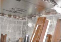
*Fire-rated Thermax® at basement ceiling*
