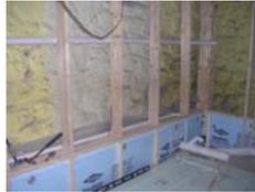
XPS “bathtub” with radiant heating
