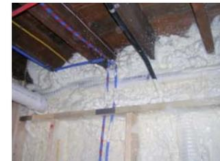
Spray foam in basement and at rim joist
