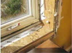
*Window with back dam and spray foam air seal*
