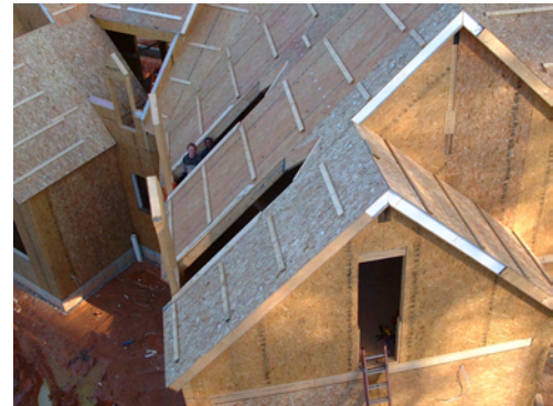
Lightweight Building 2.0 – Structural insulated panels form walls and roof, enclosing full volume within thermal envelope. (photo: Al Cobb, SIP School)
