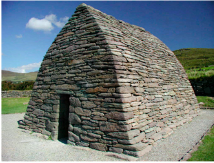
An Irish Church from 1000 AD composed of just dry-stacked rock. Simple and durable, but hardly comfortable
