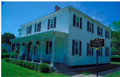
Light-weight Building 1.0 – The first frame building in Ellicottville, NY (1817) with balloon framing, non-standard wood elements and irregular spacings, fastened with both wood pegs and hand forged iron nails.
