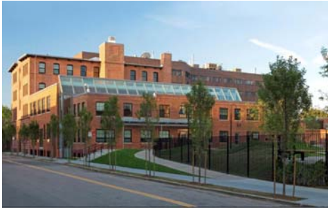
Freeze-Thaw Resistance of Clay Brick 2010.12.06
