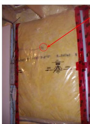
A photograph showing a yellow wafer sensor installed in a wall assembly. A red arrow points to the sensor with the text: “Wafer” sensor roughly at grade.
