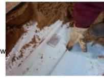
Vapor barrier over XPS with sand before slab is poured
