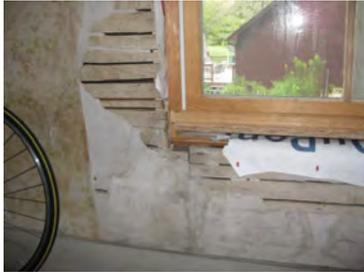
Existing replacement windows installed without flashing
