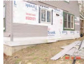
Siding removed to remediate flashing
