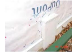
Drainage plane remediation at base of wall
