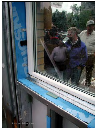
Continuous interior angle provides backdam and airseal continuity
