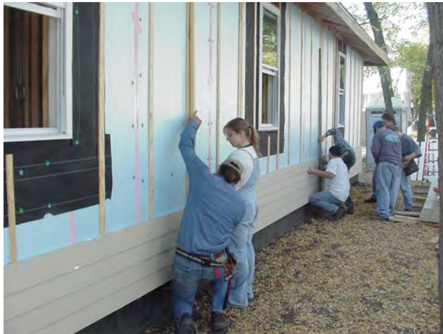
Engineered wood siding being installed over 3/8" furring strips
